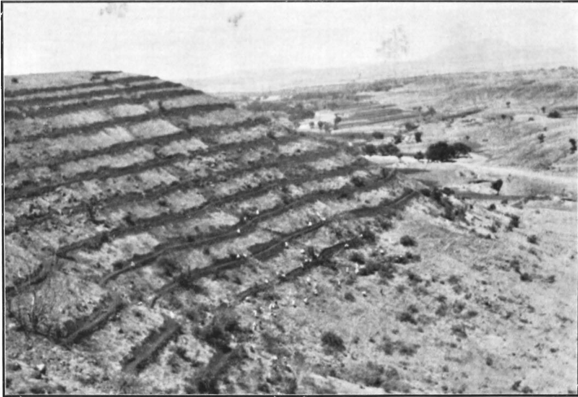
Contour trenching near Khed, Poona division. The average horizontal spacing is 24' except near the top.
