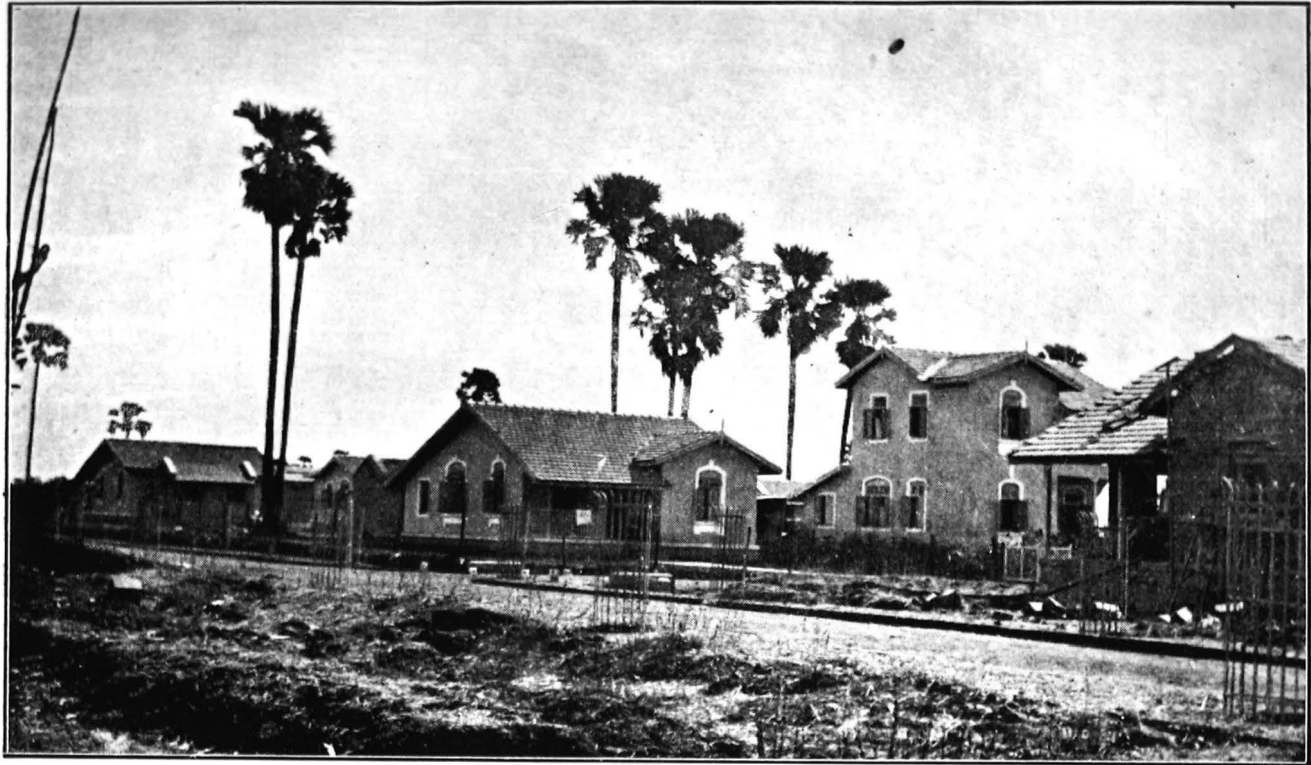
Typical cottages erected in S.S. No. 7, Khar.
