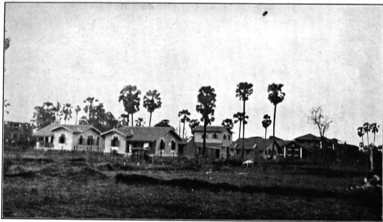
Typical cottages erected in S.S. No. 7, Khar.
