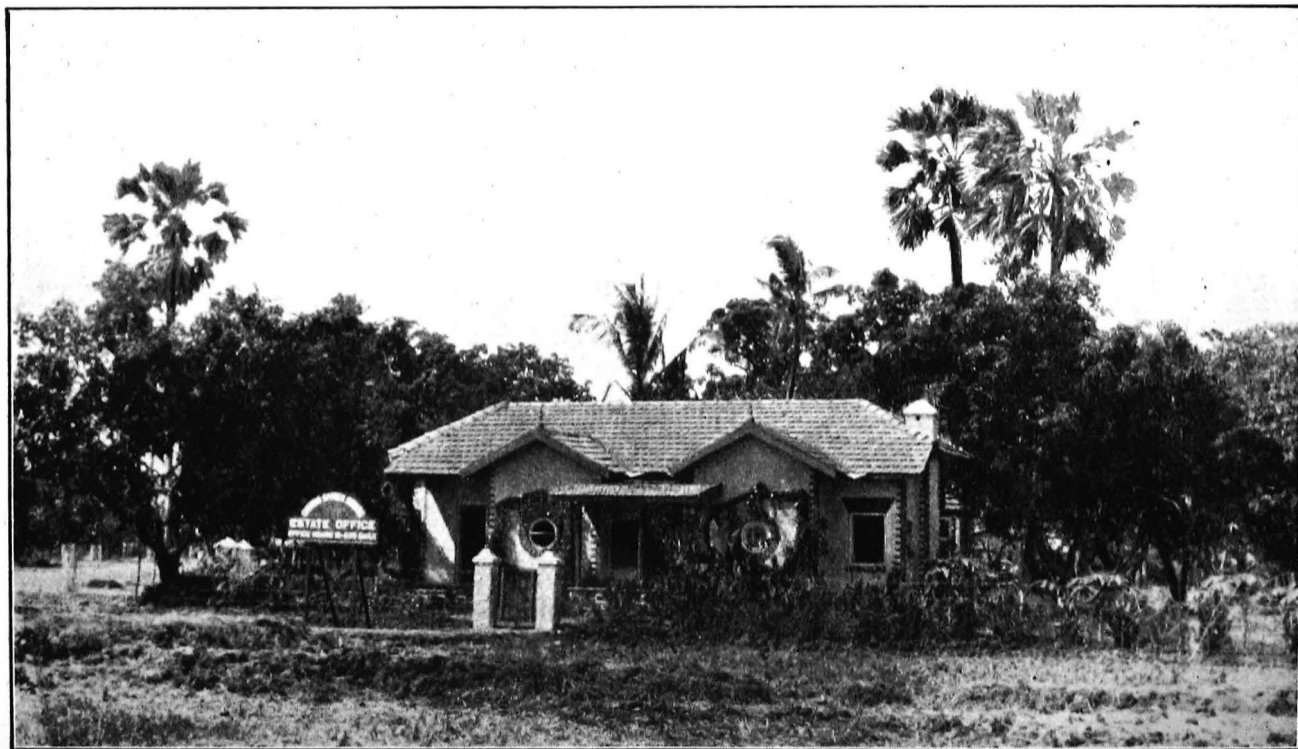
Cottage built for demonstration purposes in S.S. No. 3, Chembur Garden Suburb. For plan and details see plate D accompanying report of the Directorate for the year ending 31st March 1924.
