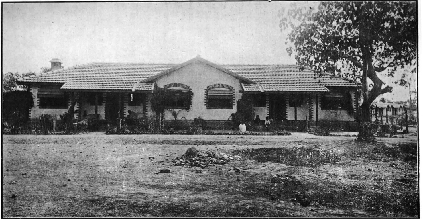
Suburban Scheme No. 3 (Chembur Section "A"). Front elevation of two semi-detached quarters type No. 5 (cost Rs. 4,350 each). Date 3rd April 1924.
