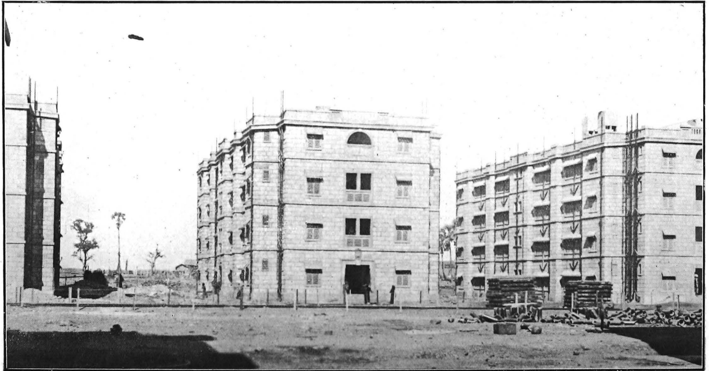
Directorate Chawls at Worli showing the open space left between each block.
