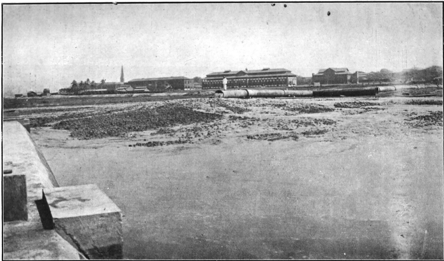
Discharge from Dredger Pipe Line at Colaba. Date 3rd February 1924.
