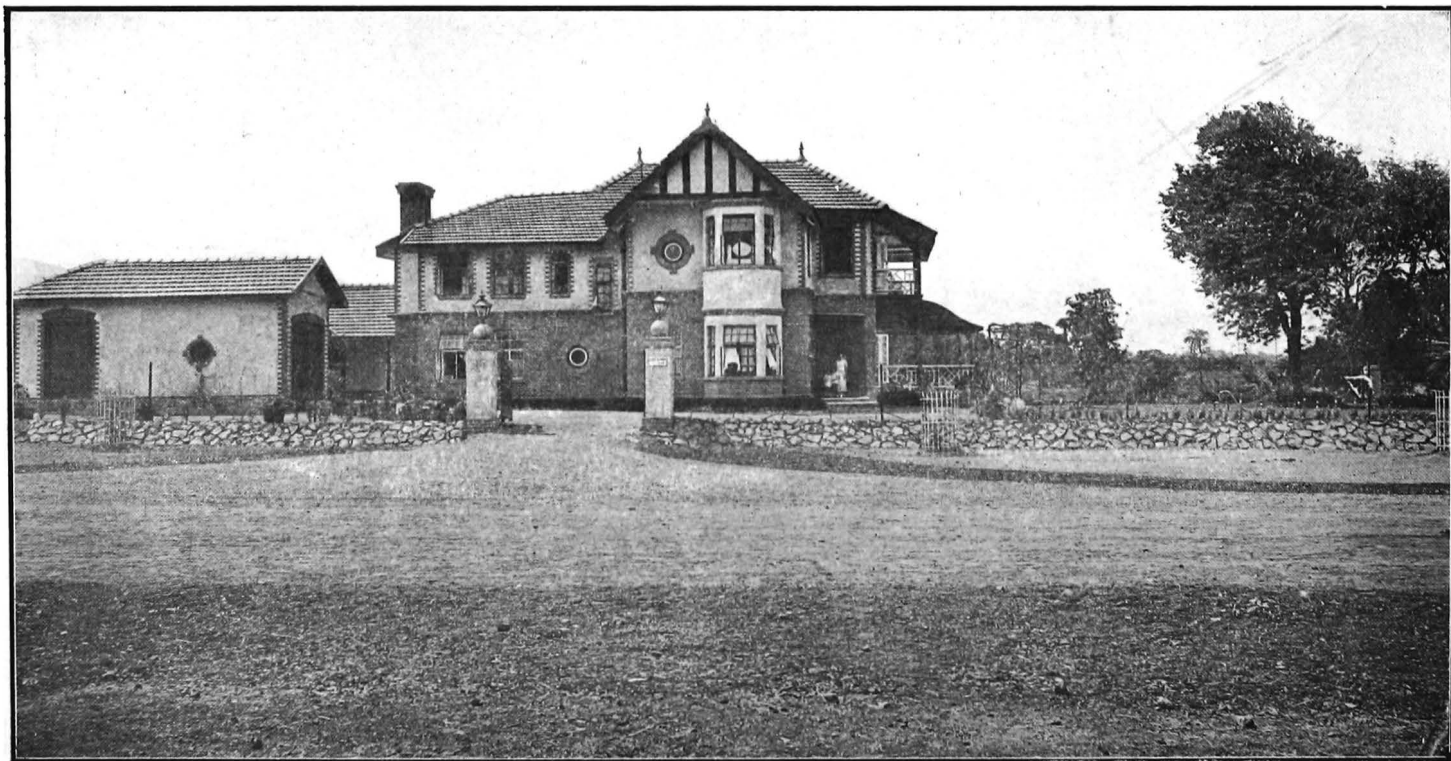
Suburban Scheme No. 3 (Chembur Section "A"). • Bungalow (cost Rs. 42,000), erected in the Garden Suburb by the Development Directorate. Date 3rd April 1924. •
