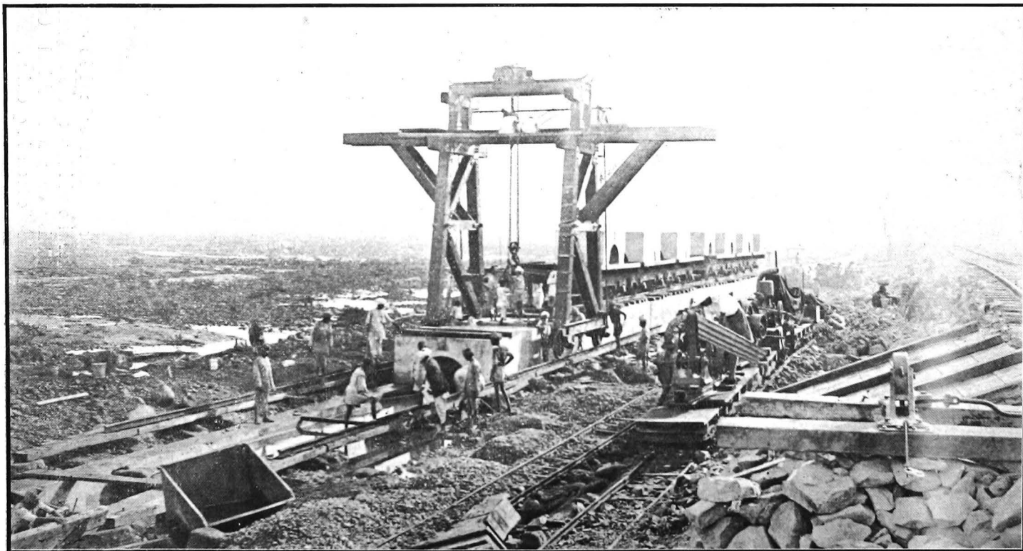
Placing 10-ton pre-cast blocks. No. 1 S. W. D. Date 27th November 1923.
