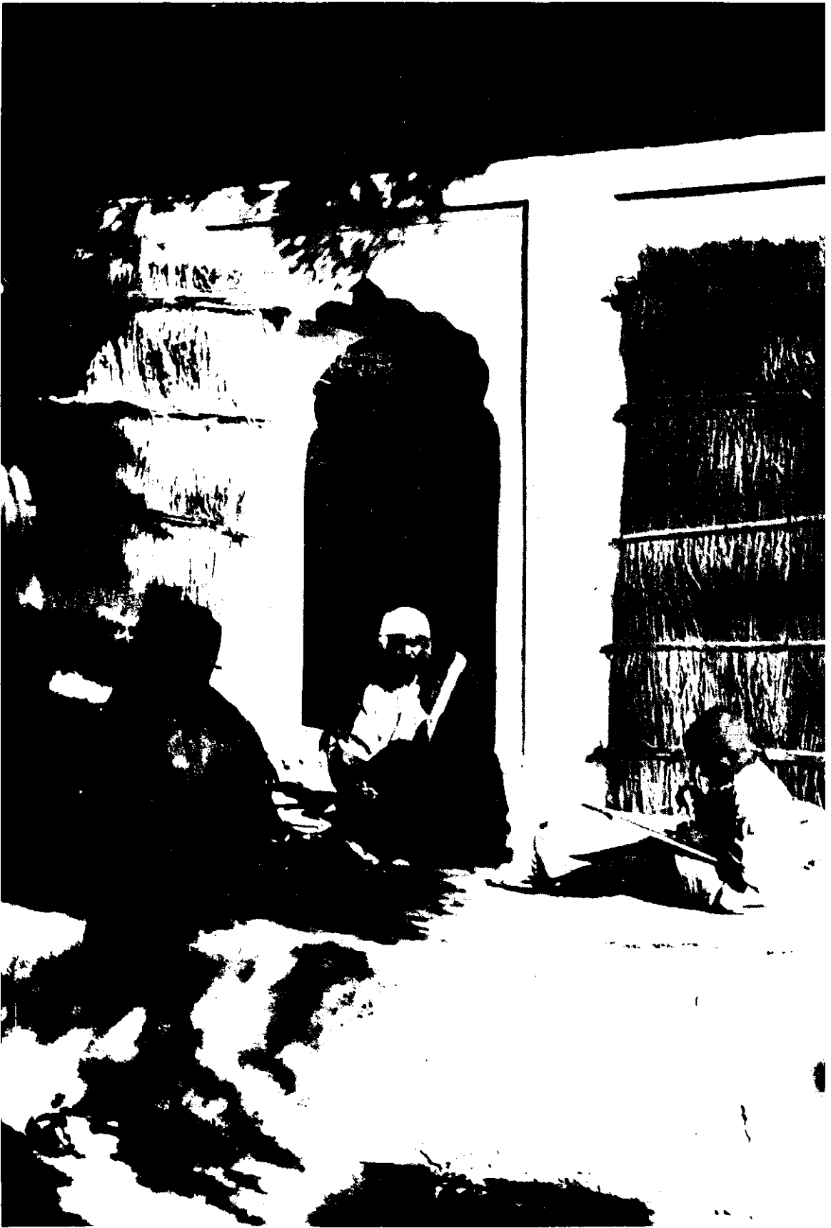
16 'Moistened fibre "tatties" hung over doors and windows cool the air but do not make it dank.'
