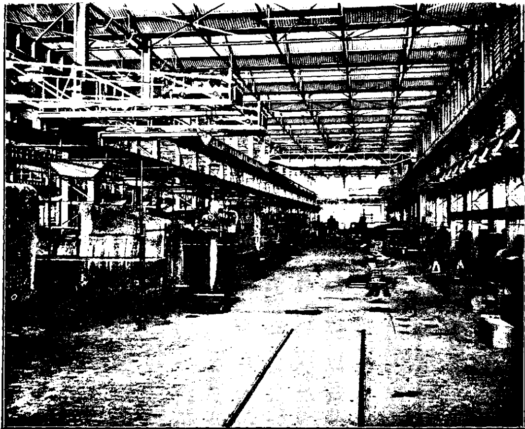
BOILER SHOP OF THE B. B. & C. I. RAILWAY LOCO WORKSHOP AT FREELANDGUNJ, DOHAD
