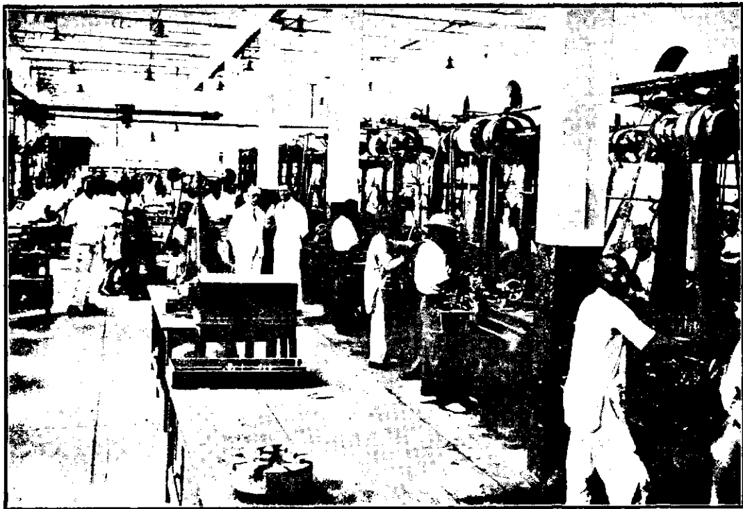
THE TOOL SECTION—AMMUNITION FACTORY AT KIRKEE (Work to very fine limits is carried out in this Section)
