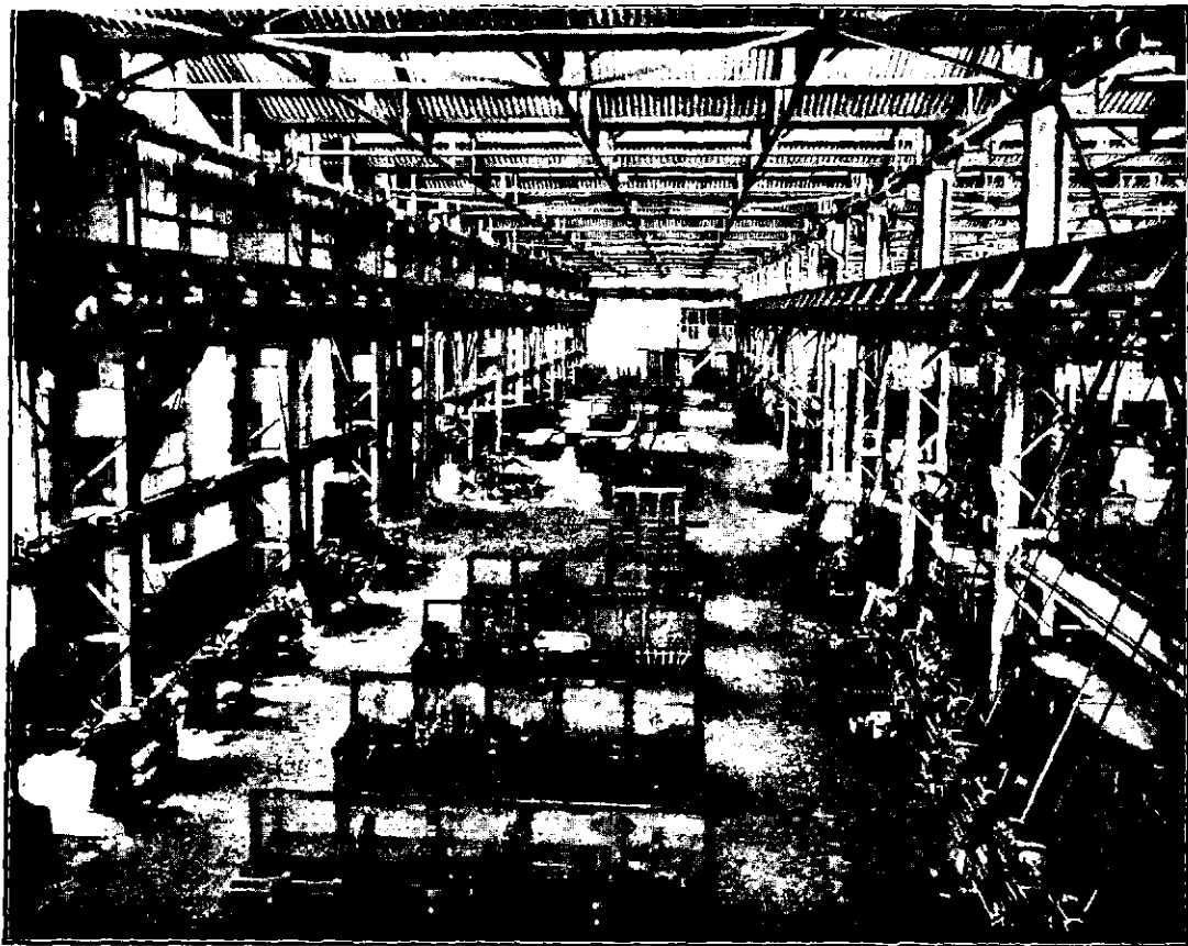
FITTING SHOP OF THE B. B. & C. I. RAILWAY LOCO WORKSHOPS AT FREELANDGUNJ, DOHAD
