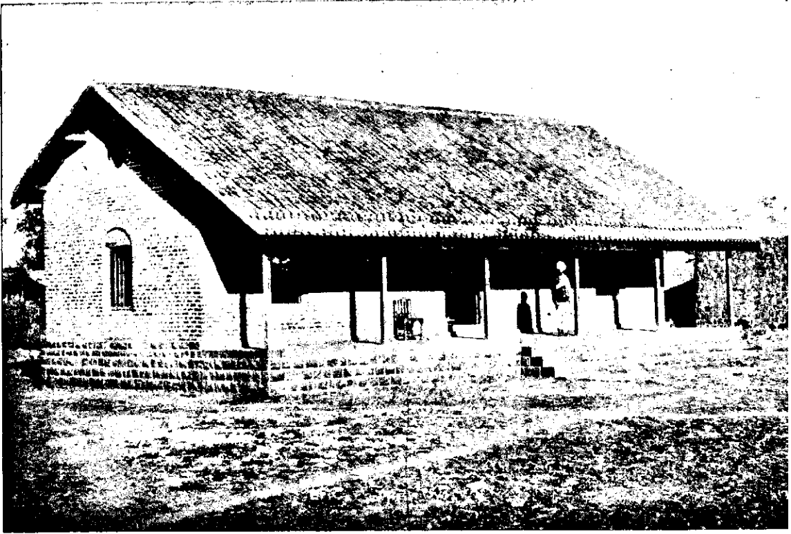
LOCAL BOARD PRIMARY SCHOOL, BUILDING AT AMNAPUR.
