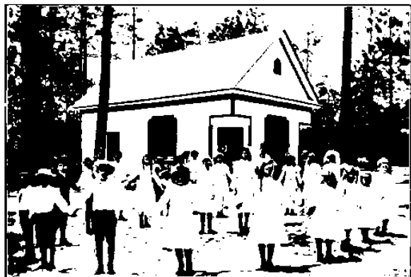
FIG. 125. A New Schoolhouse at Snow Hill, Hancock County, Georgia
