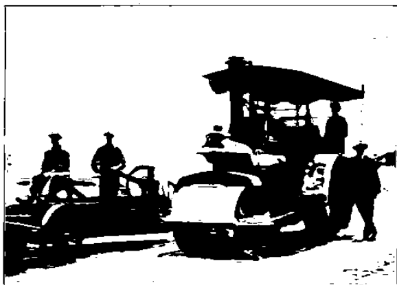
FIG. 5. A Steam Roller and a Road Scraper
