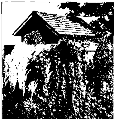
FIG. 30. Treatment of Outbuildings
