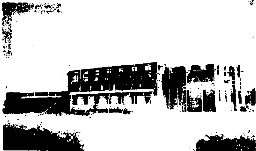
THE MAIN BUILDING UNDER CONSTRUCTION
