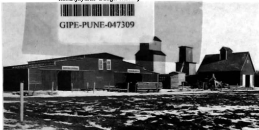
Typical elevator structure and other buildings of a farmers' elevator company.
