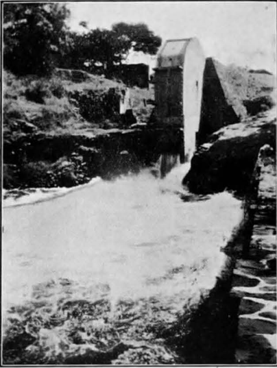
Khadakvasla Siphon Spillway, Siphon just at the point of full priming. ( Q = 150 Cs.) (I. D. R. N. 5.*)
