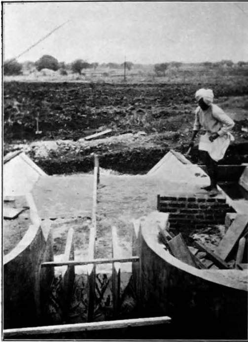
Model of Baffle-boom dissipator (Left) compared with biff wall dissipator (Right) from above fall. (I. D. R. N. 26.)*
