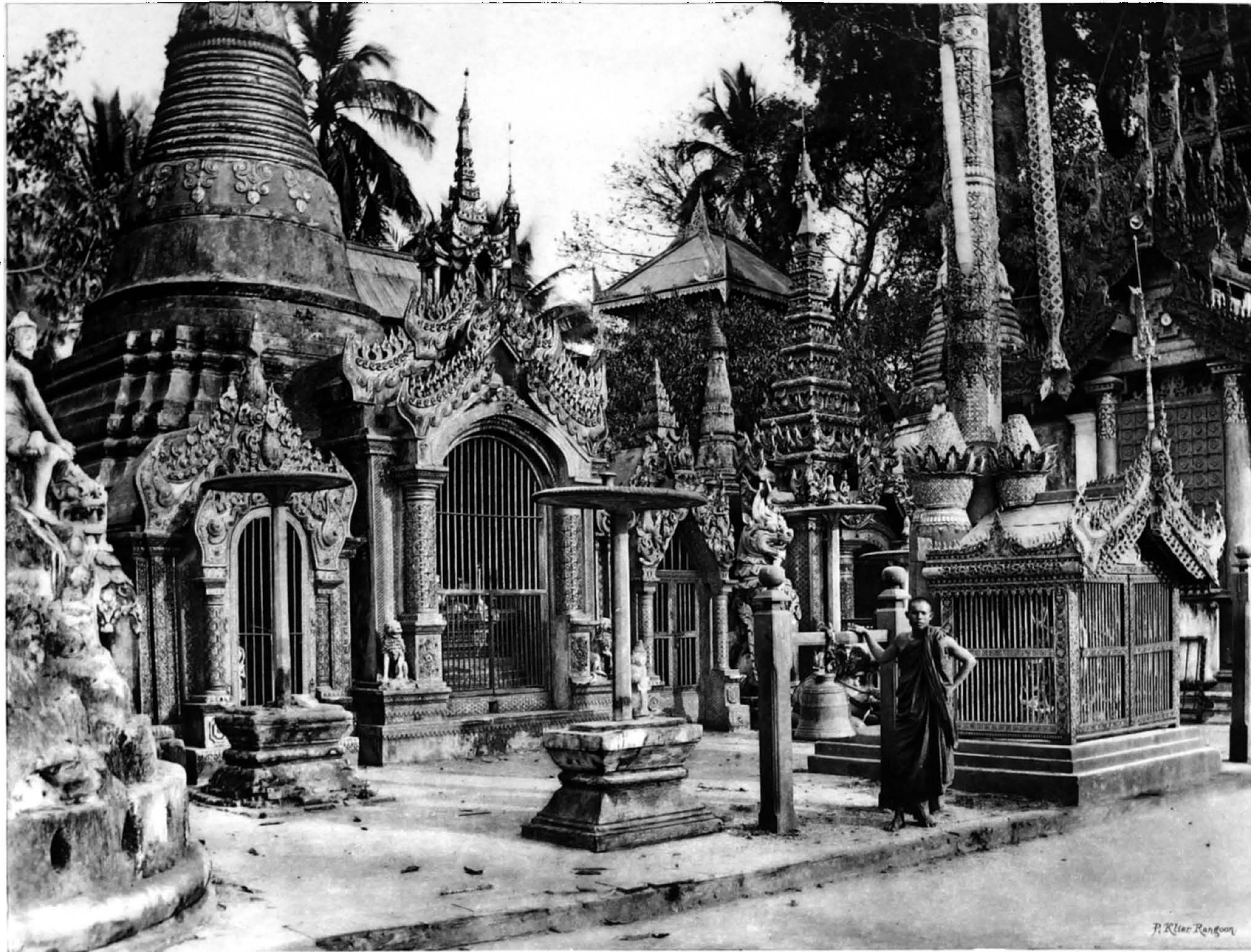
PHOTOGRAPH No. 2—ENLARGED VIEW OF SHRINE IN SOUTH-EAST CORNER,
