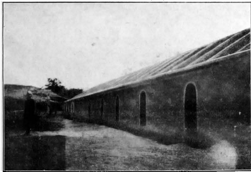
BERHAMPUR. New sleeping accommodation on right.
