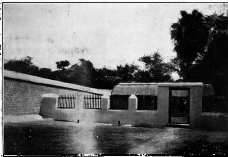
BANKURA. Showing boundary wall—Cook shed.
