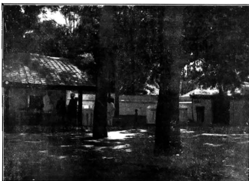
CUTTACK (T. D. L. A.) Main Rest House—Dispensary on left.
