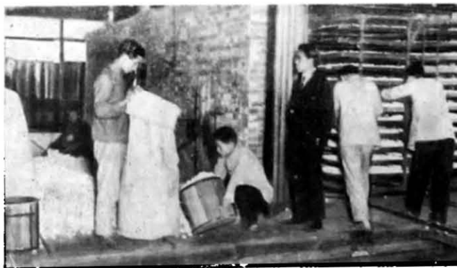
Fig. 23. Steam drying chamber (Obi-kawa system).
