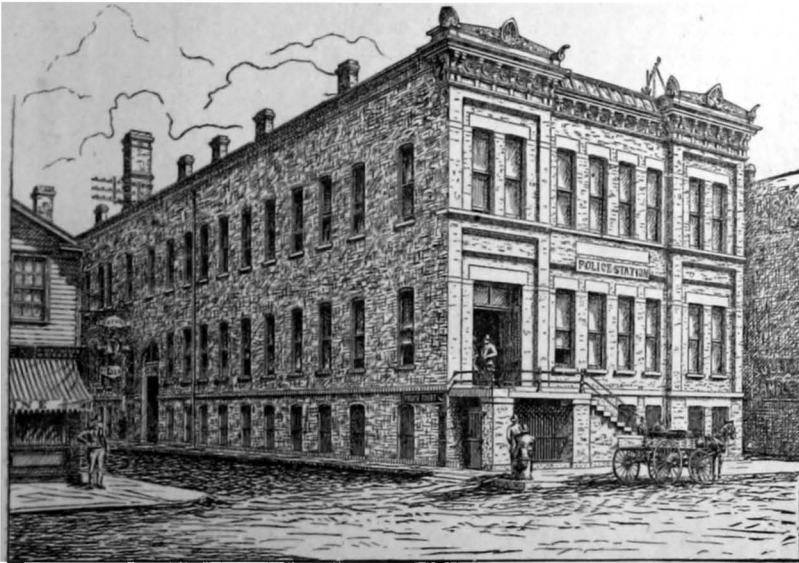
THE DESPLAINES STREET STATION.
