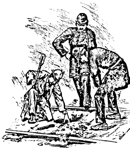
A DANGEROUS STORAGE-PLACE.
