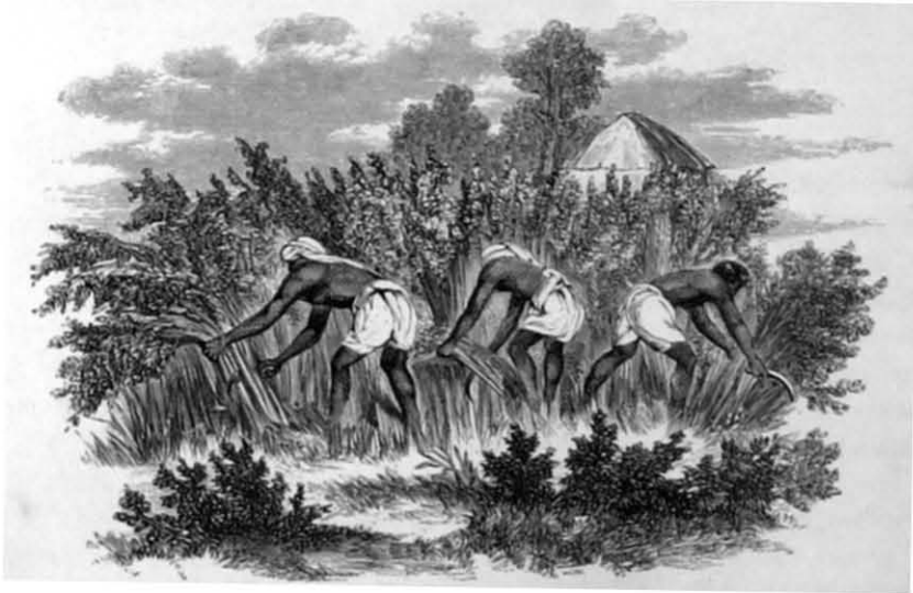
CUTTING THE PLANT.
