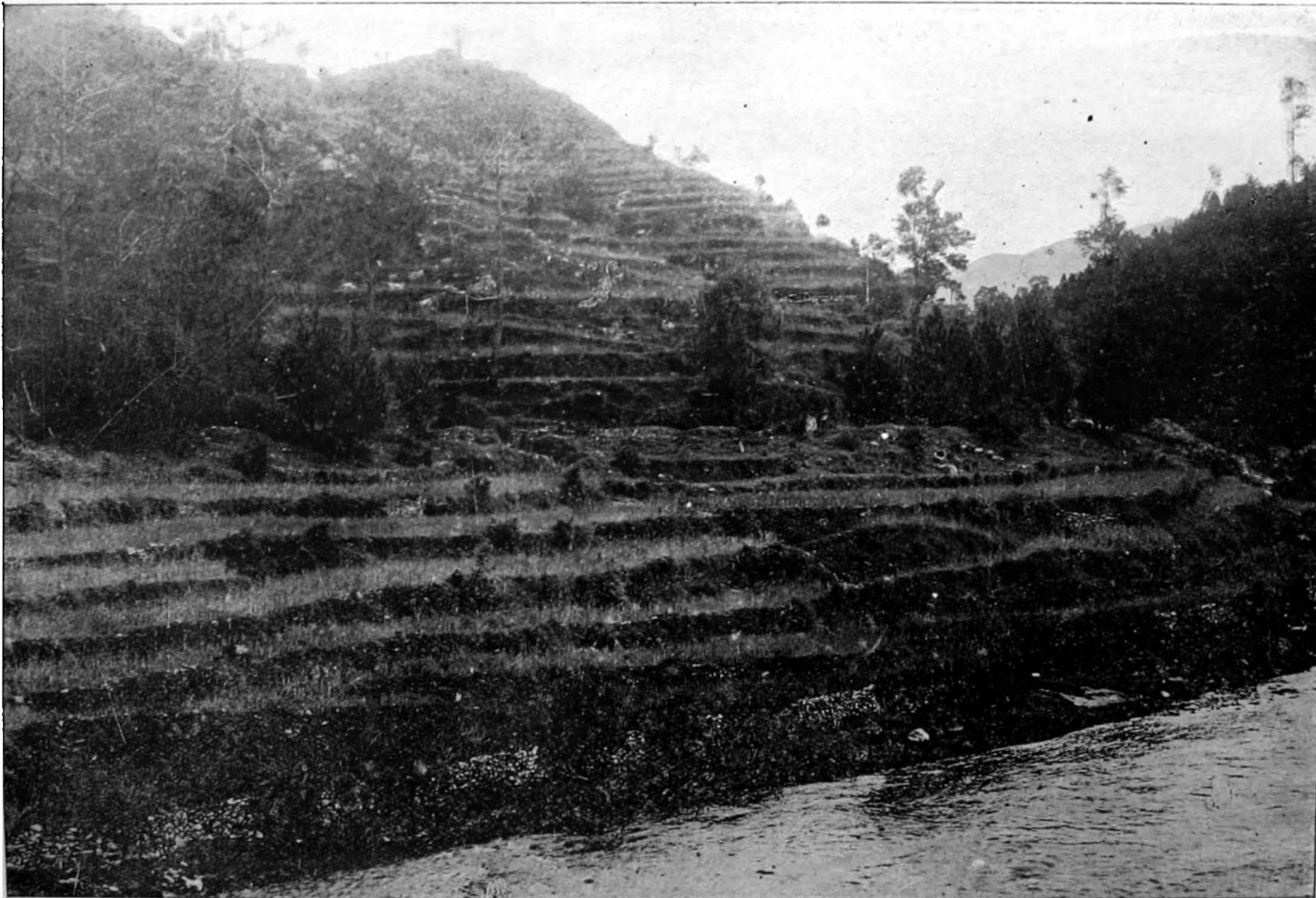
All cultivation on hillsides, except on terraces as shown above, should be prohibited. Ordinary clearances for cultivation invariably lead to erosion.
