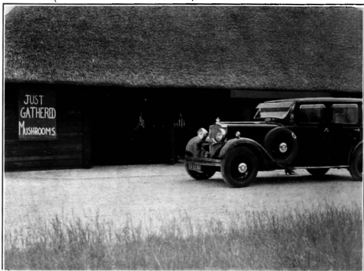
Fig. 36. Roadside kiosk for vegetables and other farm products.
