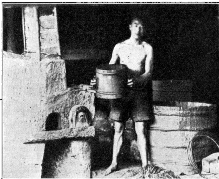
Figure 4.—Preparing tung-meal cakes for insertion in press
