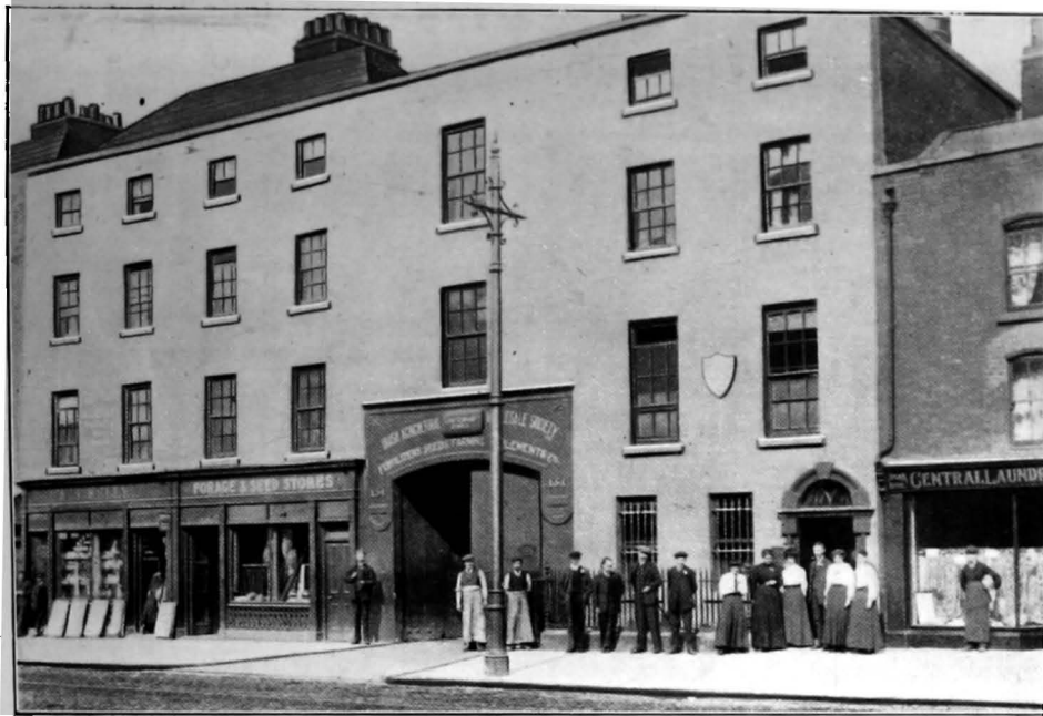
I.A.W.S. OLD PREMISES, DESTROYED BY FIRE.
