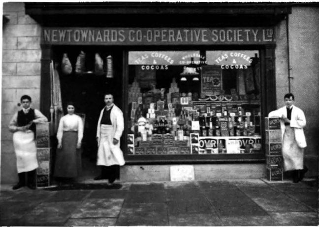
GT. FRANCES STREET PREMISES.
