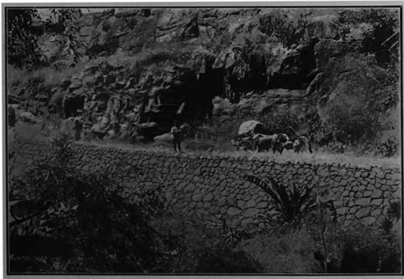
FIG. 18.—Road constructed along precipitous rocky hill side. The entire width of the road is carried on a stone construction length 110 ft., height 12½ ft.. Cost Rs. 711.
