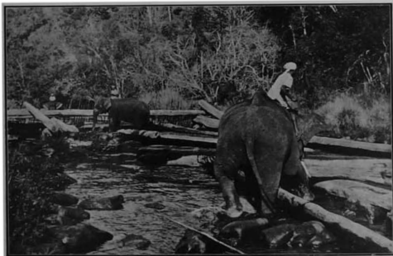
FIG. 9.—Constructing dam for floating timber with help of elephants in the Kaneri River.
