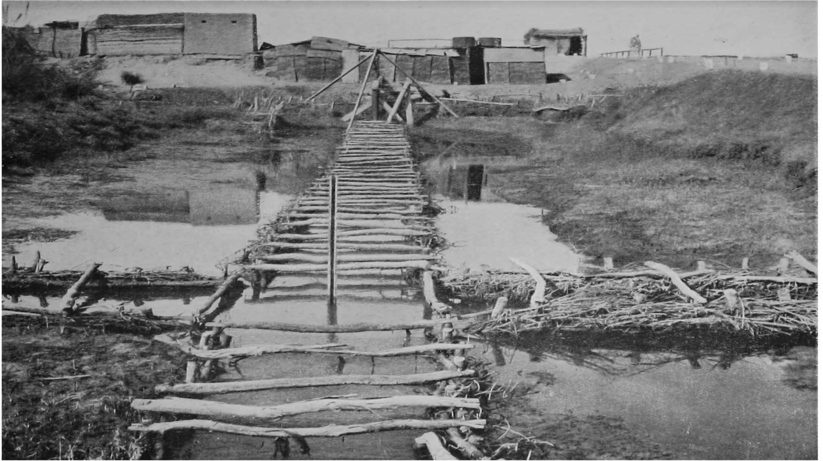
Sind : drainage difficulties owing to sand particles.
