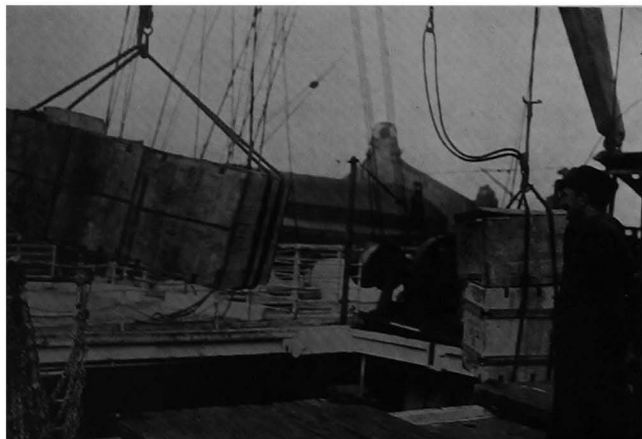
One draft has just been landed on deck. The other is swinging over the hatchway which is entirely unprotected by coamings
