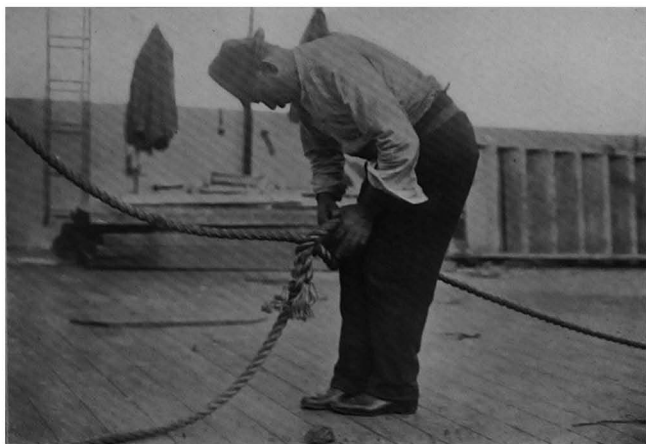
Splicing a trolley fall and a burton fall together. This is a task which requires skill and care
