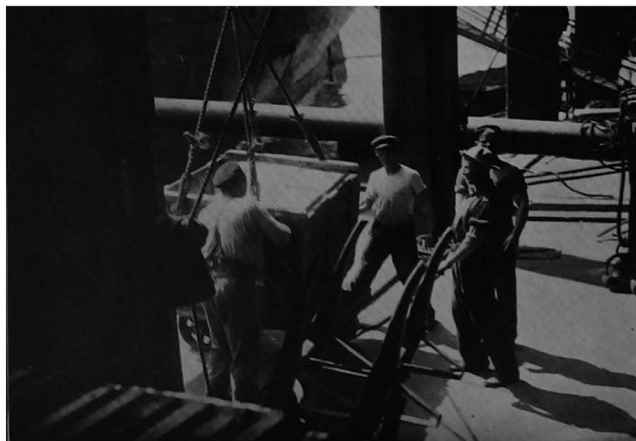
The "fruit box" as it is being landed on the pier. The pier men are standing ready with their trucks. In the background are seen a breasting-off spar (see p. 2) and a passenger gang plank
