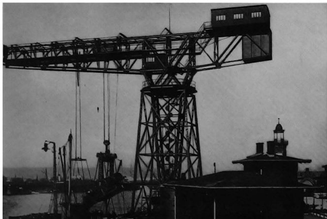
Seventy-five ton crane at the Kaiser Wilhelm Basin, Hamburg
