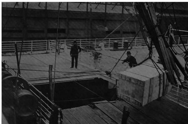
Two drafts have just cleared the hatch; one a draft of bar iron and the other a box draft. Note again the hatchway unprotected by coamings
