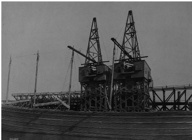
Cranes on a coal wharf, Boston harbor, unloading coal from a barge by means of clam shell scoops
