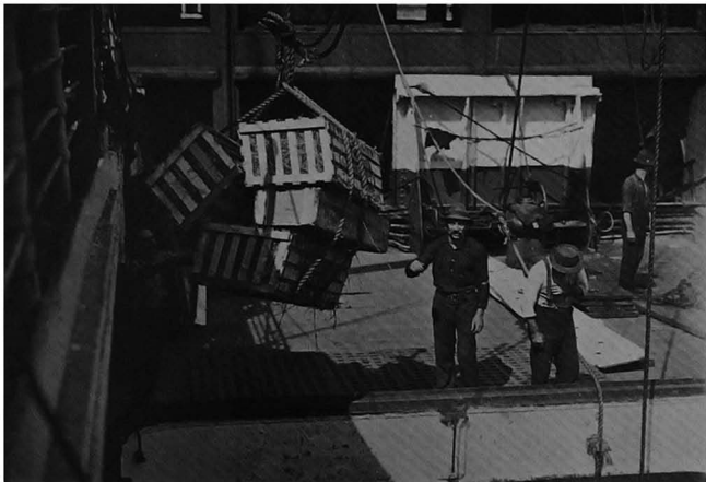
A draft of four crates has been raised from the ship's hold. In the center the gangway man is seen looking down the hatchway, giving the signal with his hand for the raising of another draft from the hold
