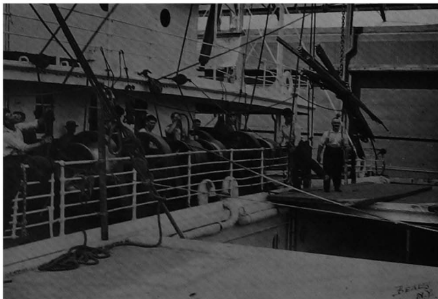
Three winches in operation. A chain sling is used in lifting the draft of bar iron. The draft is now high enough to be swung athwart the ship and lowered onto the pier. Note the unprotected hatchway
