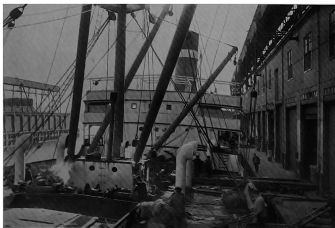
Discharging jute from an East Indian steamer at a Boston pier. Note the use of skids, or "stages," and the arrangement of booms and gear
