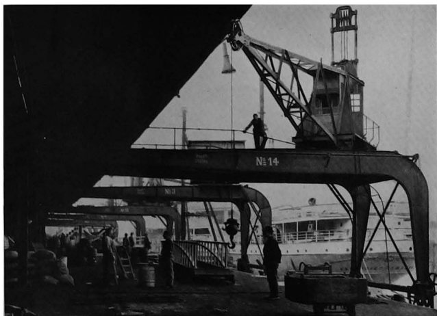
Moveable electric cranes on the Versmann quay, Hamburg
