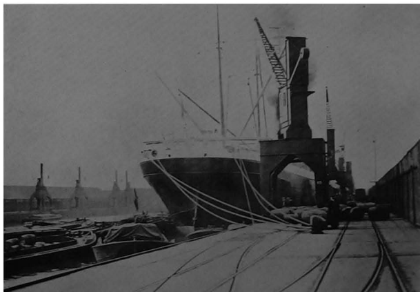
View at the Tilbury Docks, London, showing the temporary storage sheds, the hydraulic cranes, and the railroad tracks on the quay. The very large ships of recent construction which sail to London use the Tilbury docks
