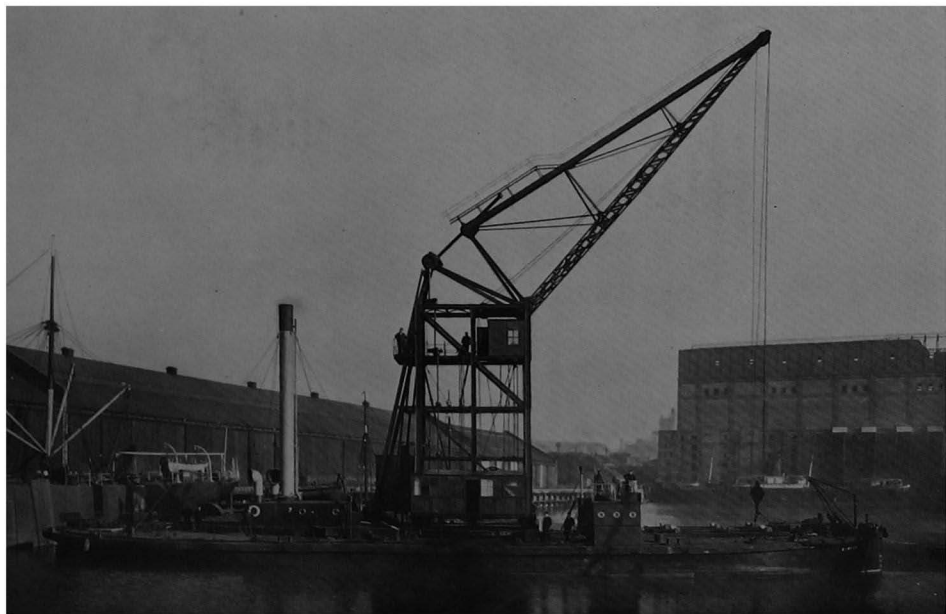
Floating crane "Samson," Liverpool. Capable of dealing with loads up to thirty tons in weight
