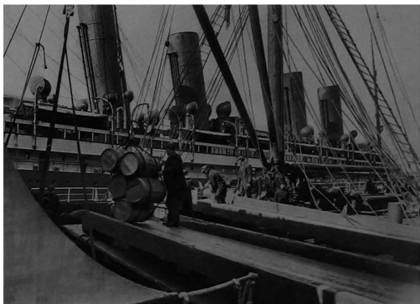
Loading at a Boston pier. The skids, or "stages," extend to the verge of the open hatchway. In the background lies the "Kronprinzessin Cecilie" interned during the war
