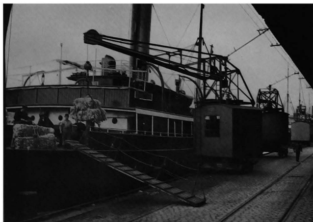
Electric trolley cranes on the Kaiser quay, Hamburg
