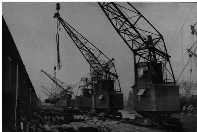
Moveable electric cranes on the Kuhwärder quay, Hamburg
