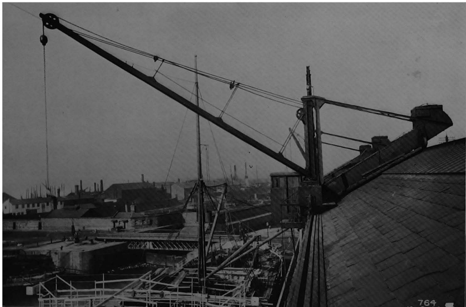
Roof crane for discharging goods from vessels, Liverpool. Capacity thirty cwts.
