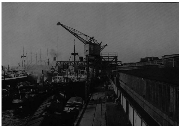
Moveable cranes, showing railroad tracks beneath and platform of the pier shed. Along the wall of the shed and at the edge of the pier are seen the tracks on which the cranes are moved
