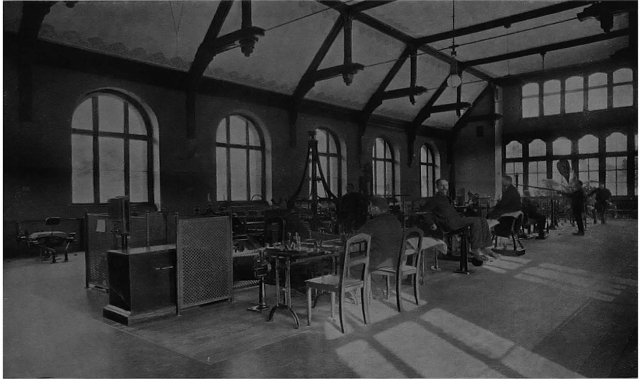
BEEELITZ SANATORIUM (BELONGING TO THE BERLIN PENSION BOARD)—ZANDER HALL FOR MEDICO-MECHANICAL APPARATUS.
