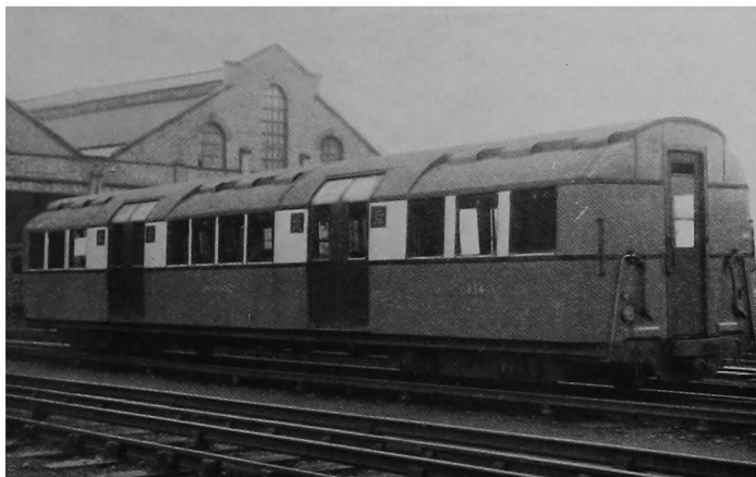
Standard tube railway car with automatically-operated doors.
