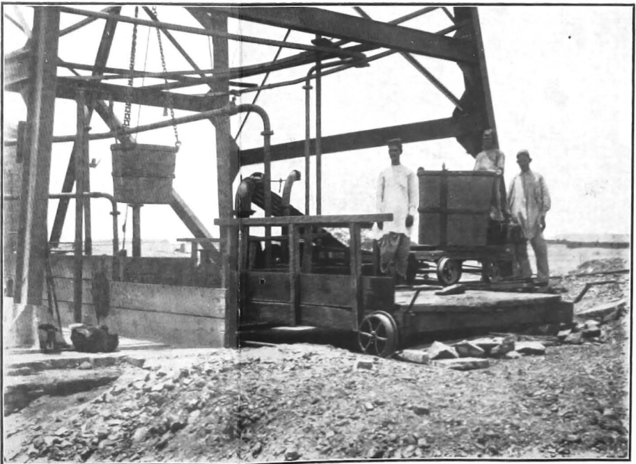
Trolley Covering Top of Sinking Shaft.
