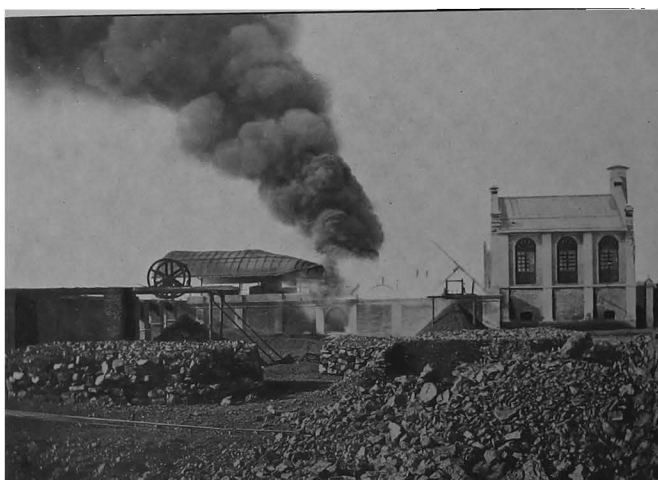
No. 17 Pit during the progress of the fire.
