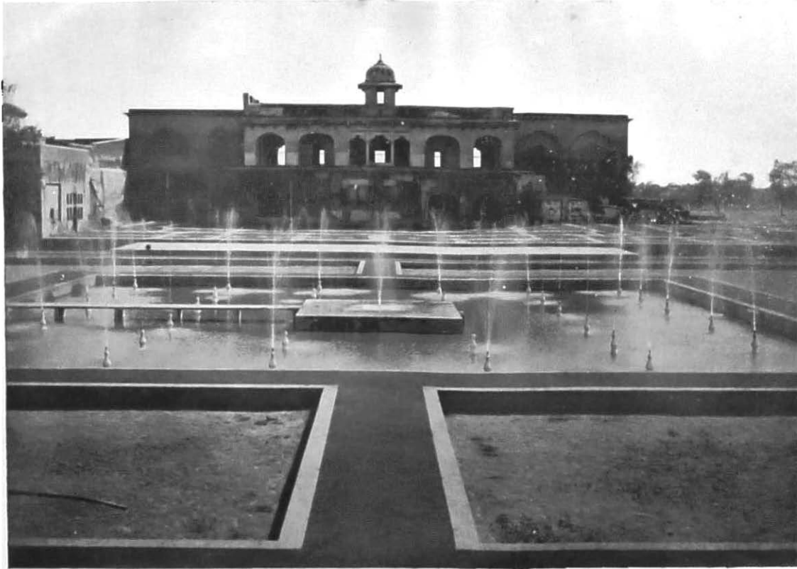
NEWLY RESTORED CAUSEWAYS AND FOUNTAINS IN JAHANGIR'S QUADRANGLE, LAHORE FORT.
