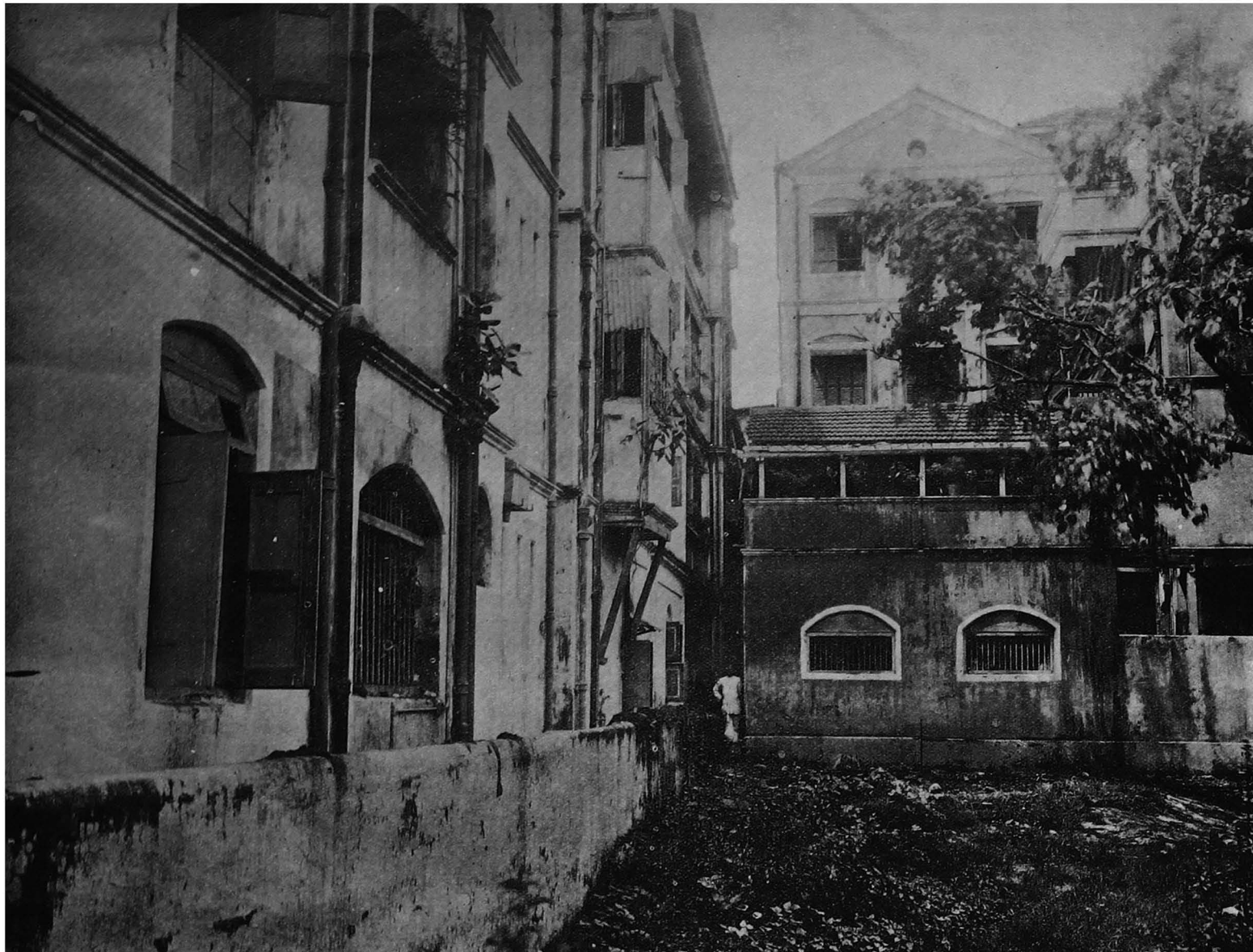
Nearer view of the houses on the right of Photo No. 5, showing the narrowness of the rear open space between the existing back to back houses. On the
