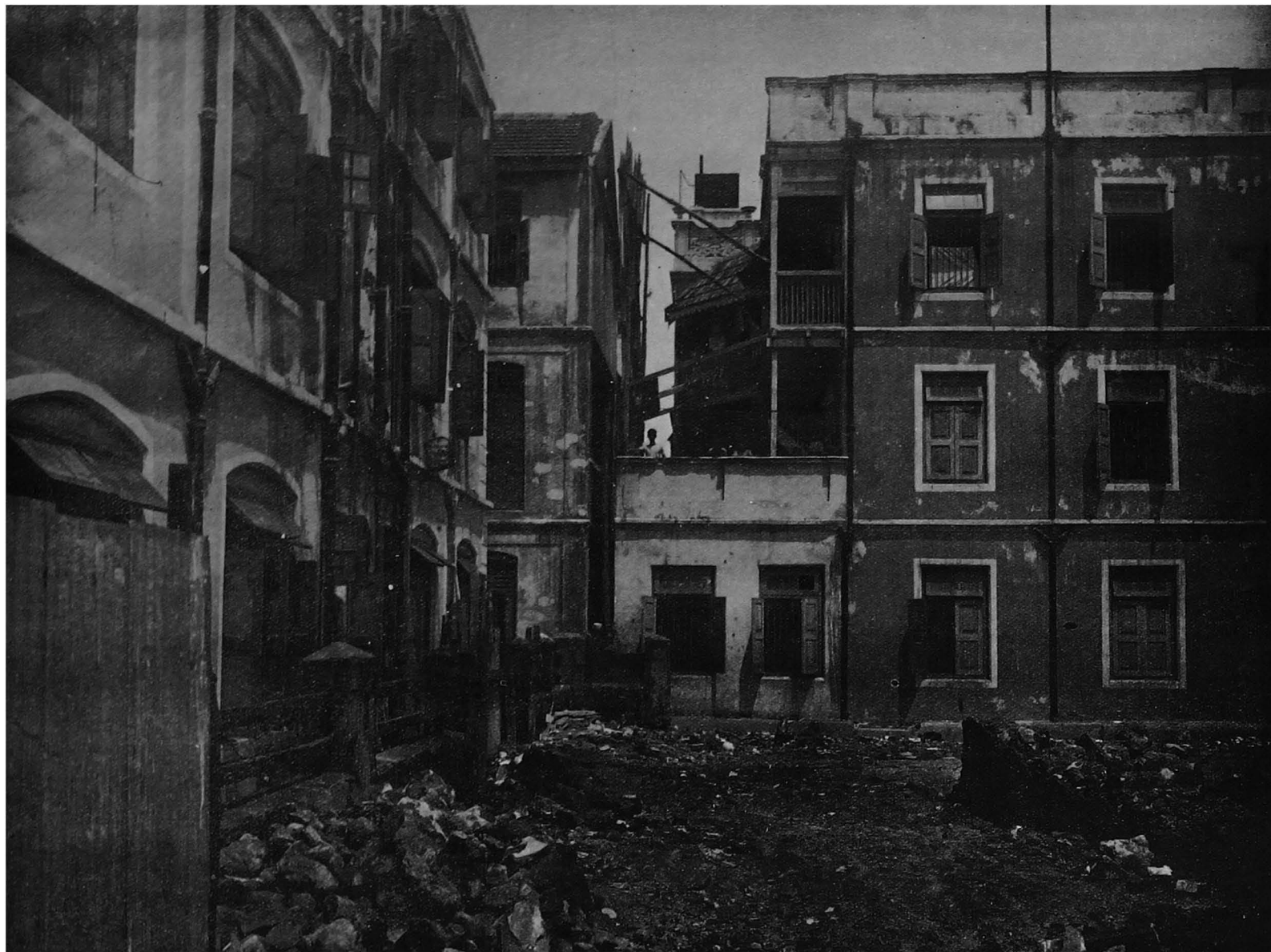
Another site yet to be built on in the group of houses shown in Photos 1, 2 and 3. Characteristics as in No. 2; most of the rooms in surrounding houses will be deprived of good light and ventilation when the site is built on. Narrow gully between ground floor building and adjacent house in the centre. Screen erected
