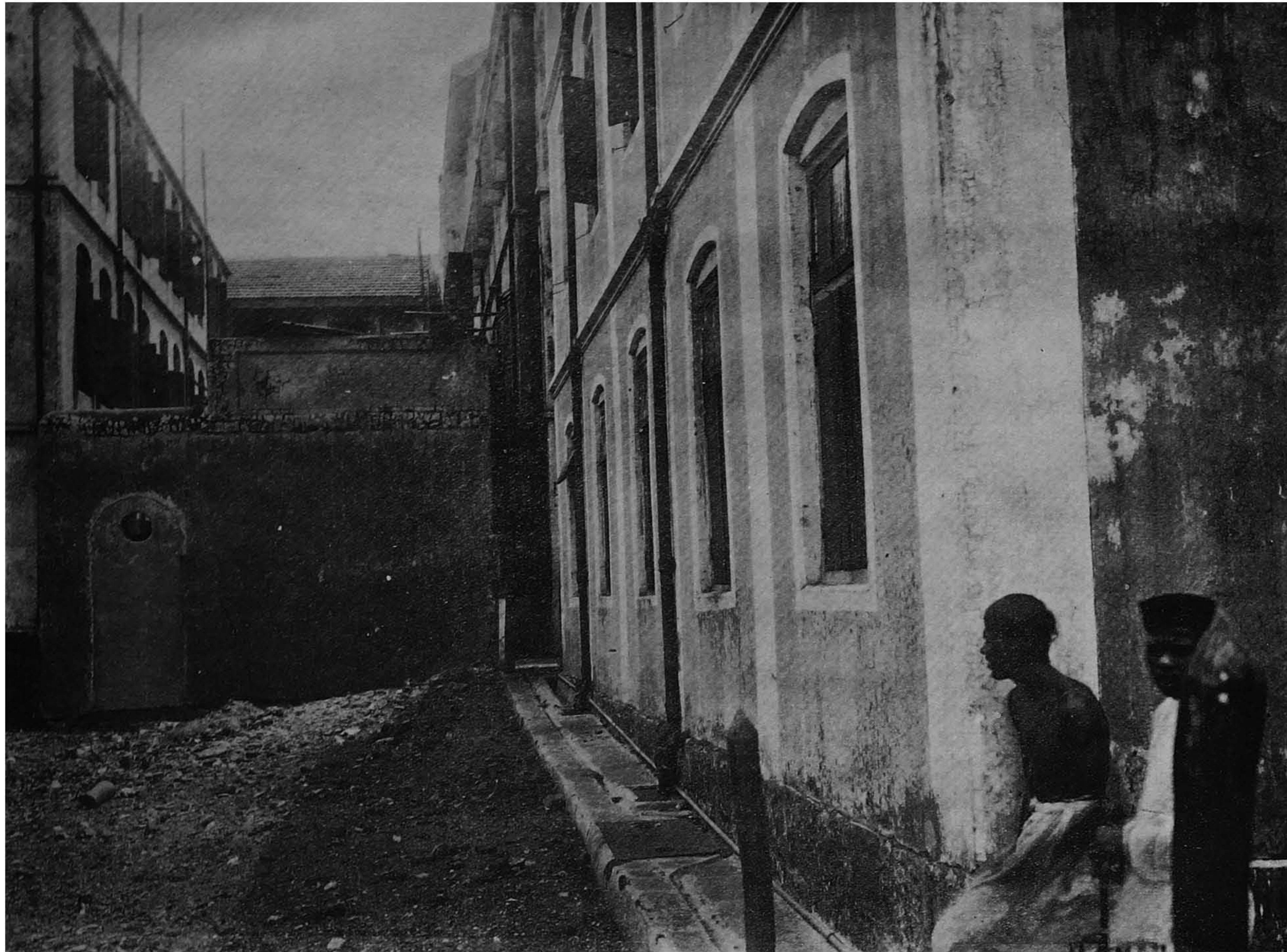
Nearer view of stable shown in Photo No.2, showing end of new upper wall blocking windows on the right. The wall is to be built up so as to block the windows
