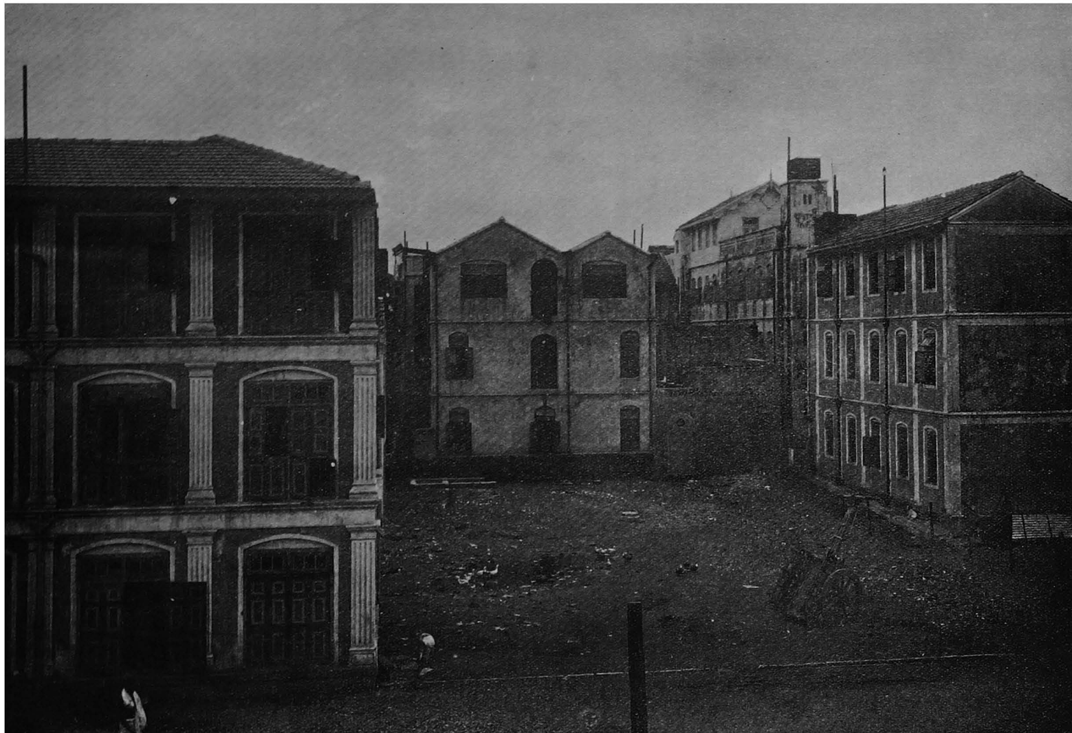
Vacant house site shortly to be built upon behind houses shown in Photo No. 1. Surrounding houses built up to within a few feet of this site with very narrow gullies between them. The low building in the background is a ground floor stable on which upper storeys are being constructed with a blank wall within 2ft. of the windows of the next building which hitherto got good light and ventilation over the top of the stable. The windows abutting on the site yet to be built on will probably be similarly obstructed by the walls of new buildings within a few feet of them.
