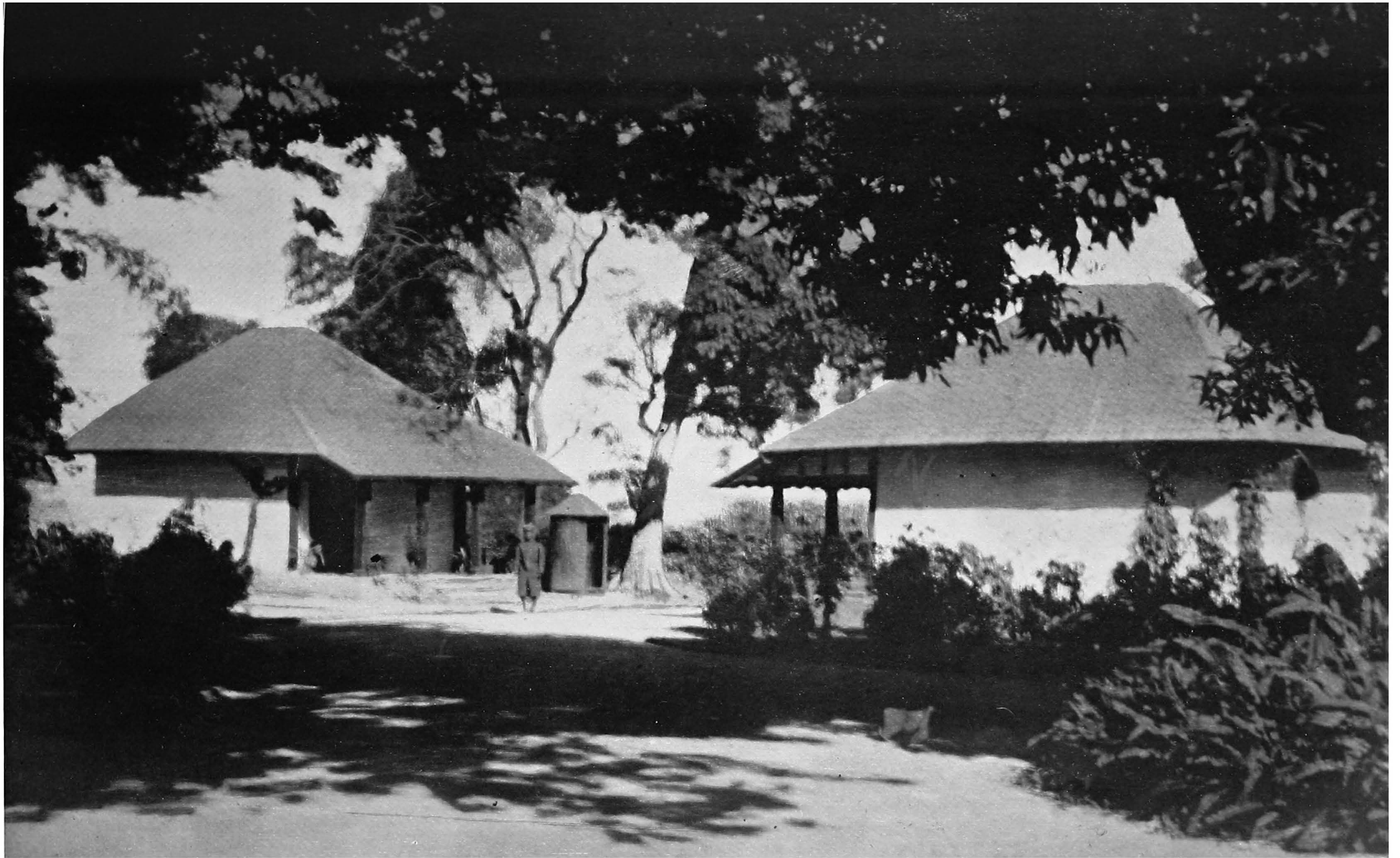
Gate House, Government House, Ranchi.
