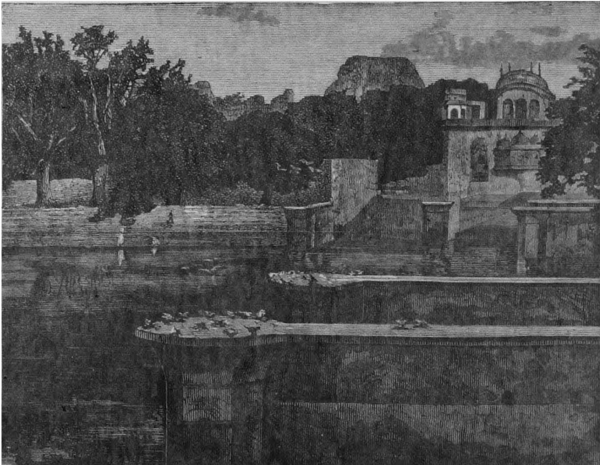
TANK AT DEEG.
