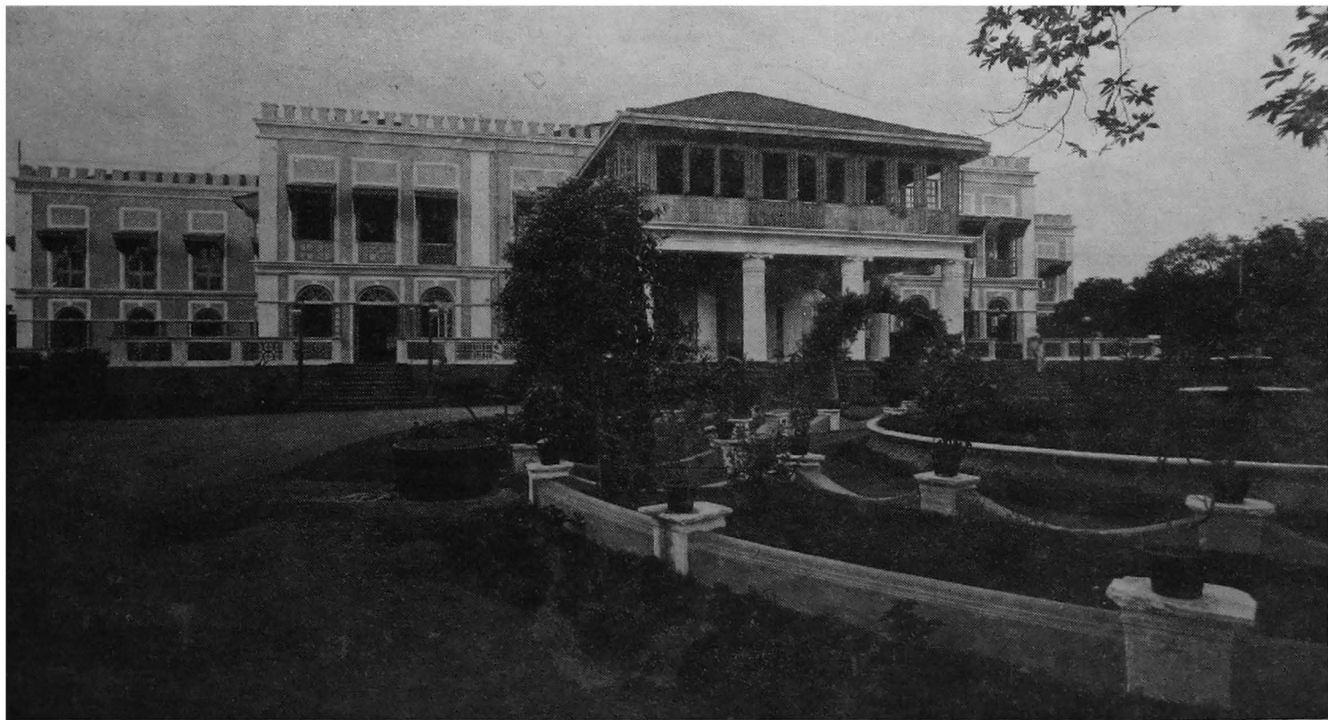
The School—Front view.
