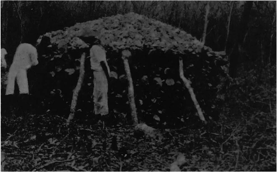
4. Burning limestone to make lime.
