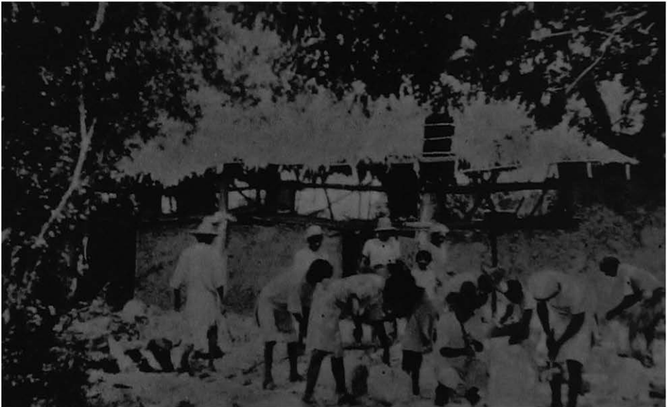
5. Fagina : work on the new school building.
