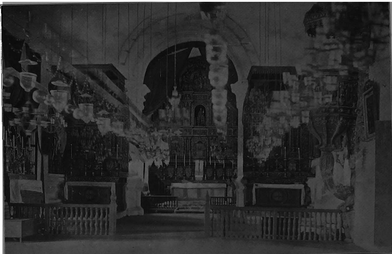
INTERIOR OF THE OLLUR CHURCH.
