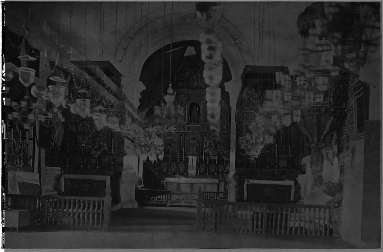
INTERIOR OF THE OLLUR CHURCH.
