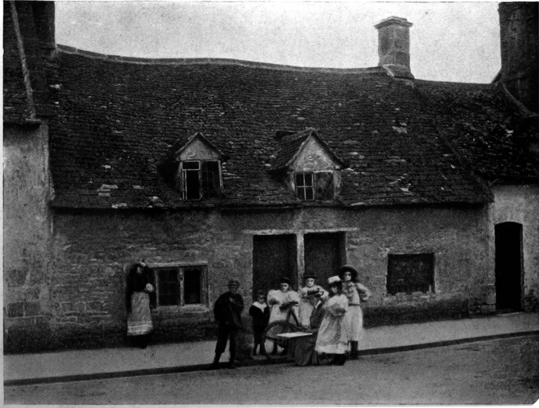
Derelict Cottages in Camden High Street.
