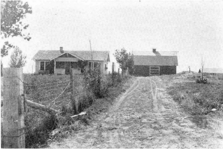
Figure 26—A well-constructed set of farm buildings on the Round Butte subdivision.
