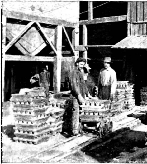
BULLION AT THE AMERICAN SMELTER, LEADVILLE, COLORADO
