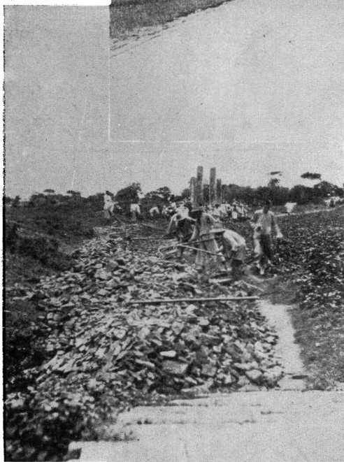
Left. Working on Broken Brick foundation
