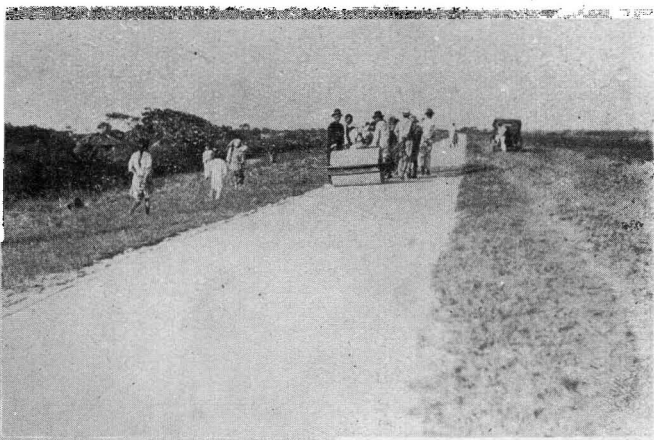
Right-workmen in process of finishing a part of the Kiangsu Section
