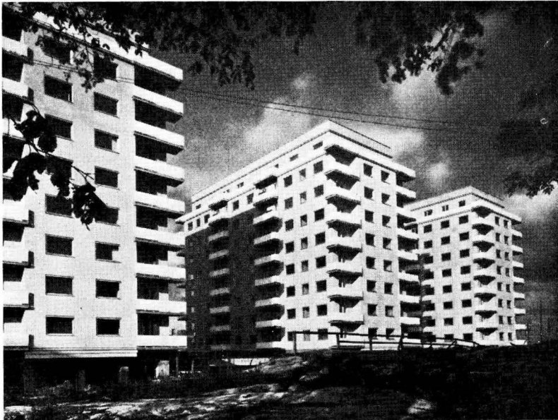
FIGURE 26.—MODERN FLATS IN STOCKHOLM.
