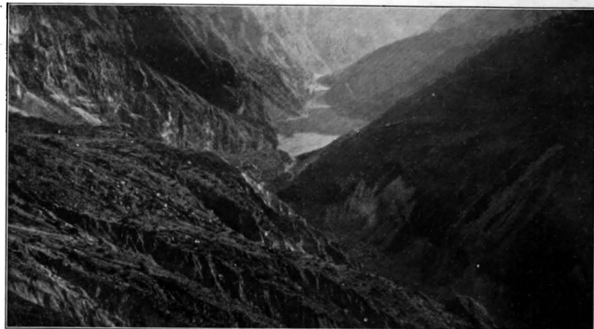
Gohna Tal looking east showing in foreground the continual heavy erosion of the old slip debris. Slip debris also seen on far bank with breach in the centre.
