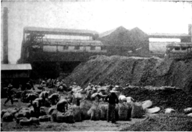
FIG. 93.—Loading coke into straw bags by hand at the plant of the Tokyo Gas Company.
