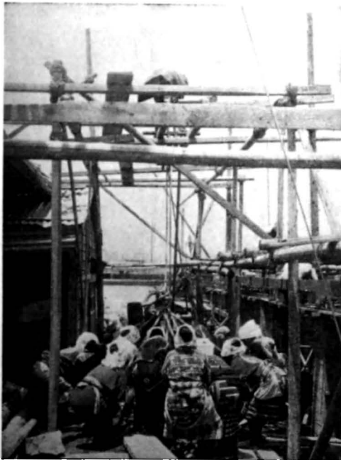
FIG. 90.—Driving piling by hand for a reinforced concrete factory building, Tokyo.
