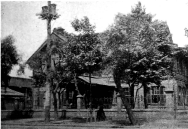
FIG. 118.—The headquarters of the General Federation of Japanese Labor are in an old Unitarian church in Tokyo.
