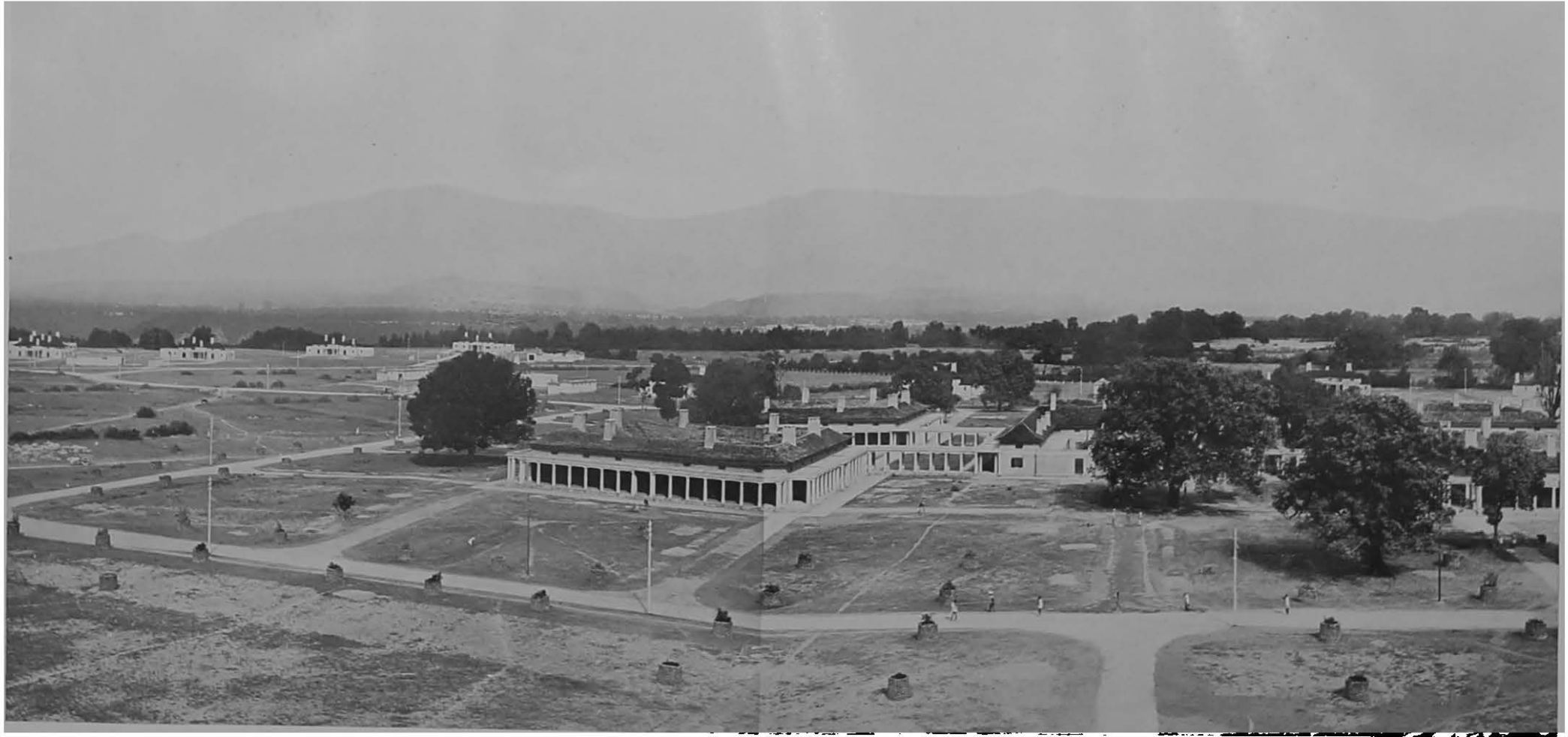
General view of the Hostel and Quarters, Railway Staff College, Dehra Dun.
