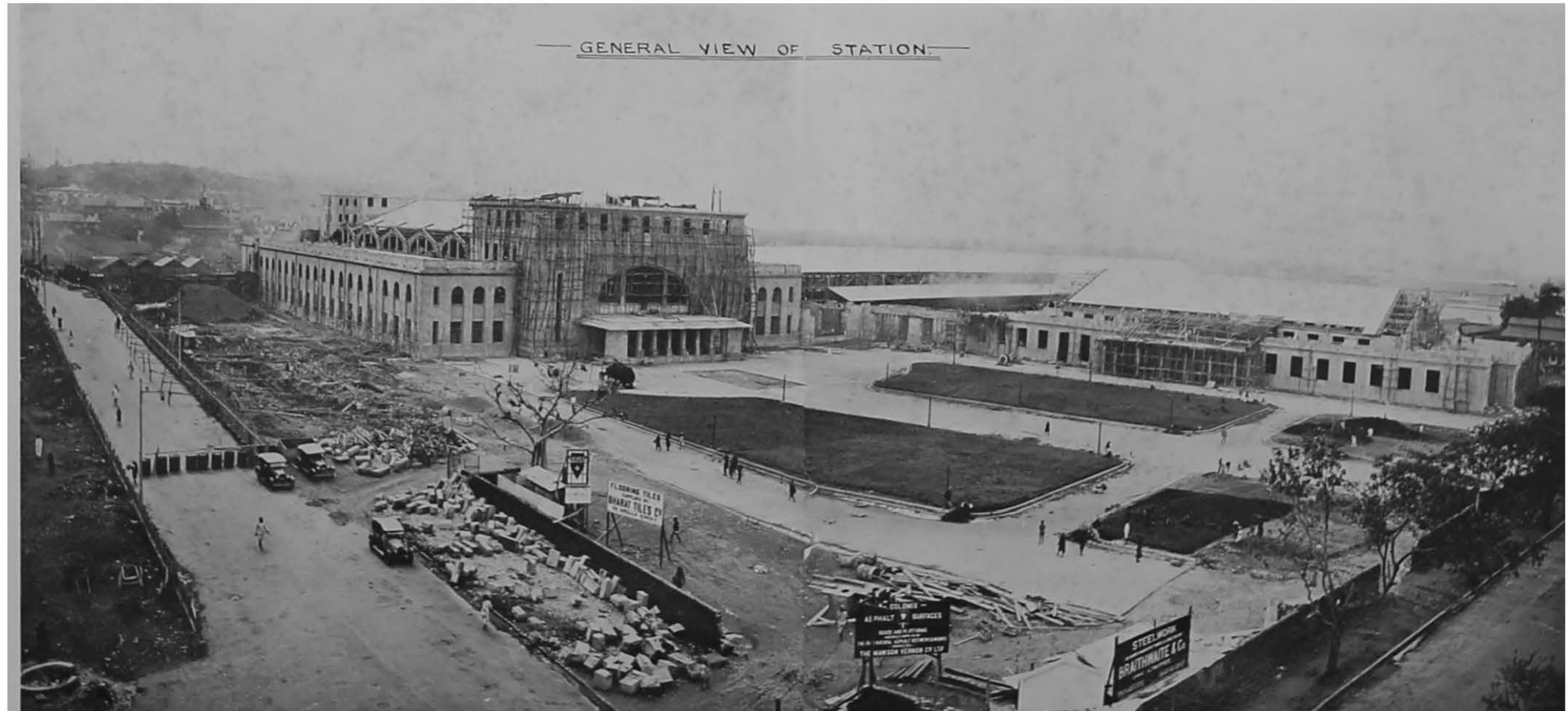
Bombay Central Station—construction in progress.
