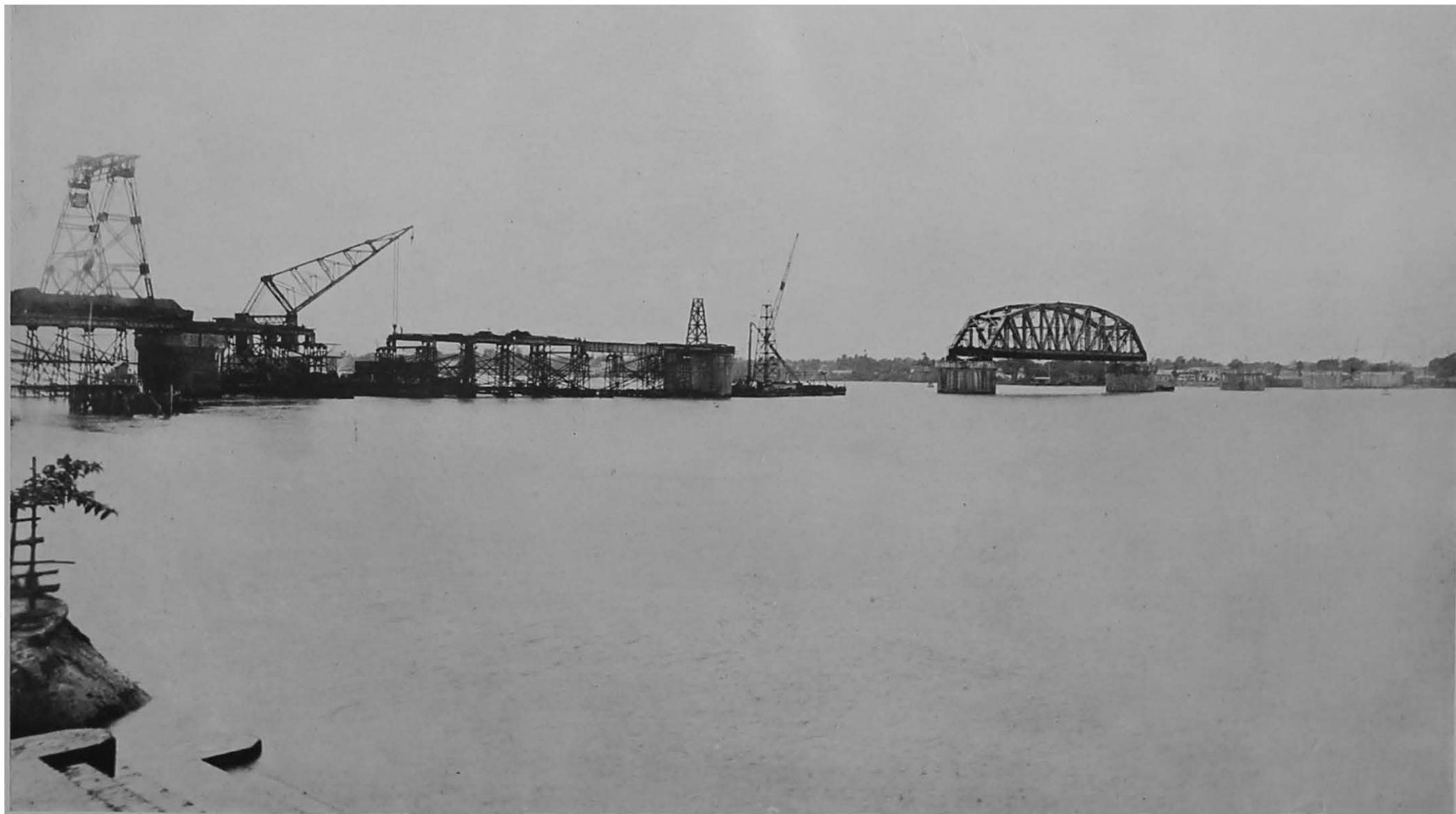
Bally Bridge—First span in position.
