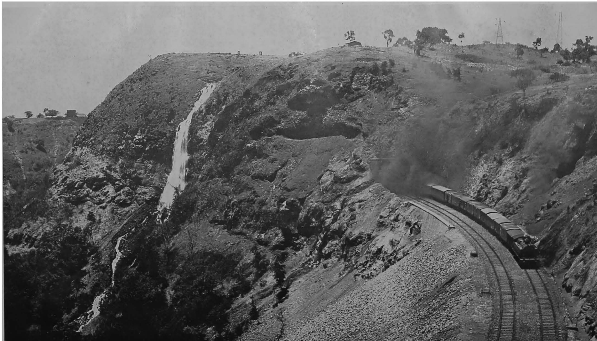
Bhore Ghat—View from the top of Tunnel No. 26.
