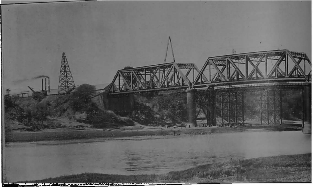
The rebuilding of the Par Bridge—Bombay, Baroda and
