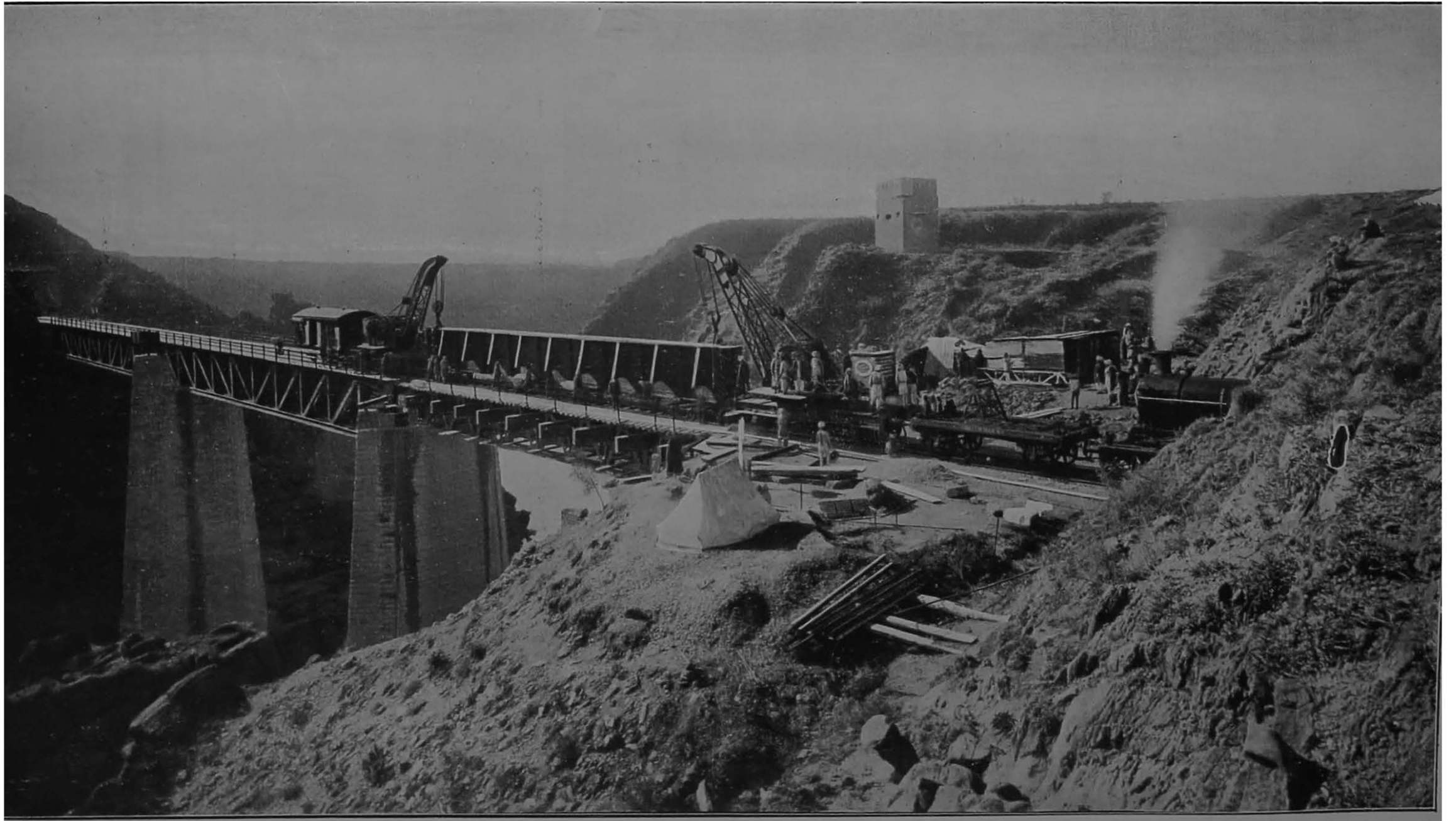
Substitution of a "Trough" Plate Girder span under traffic on the Kurang Bridge.—North Western Railway.
