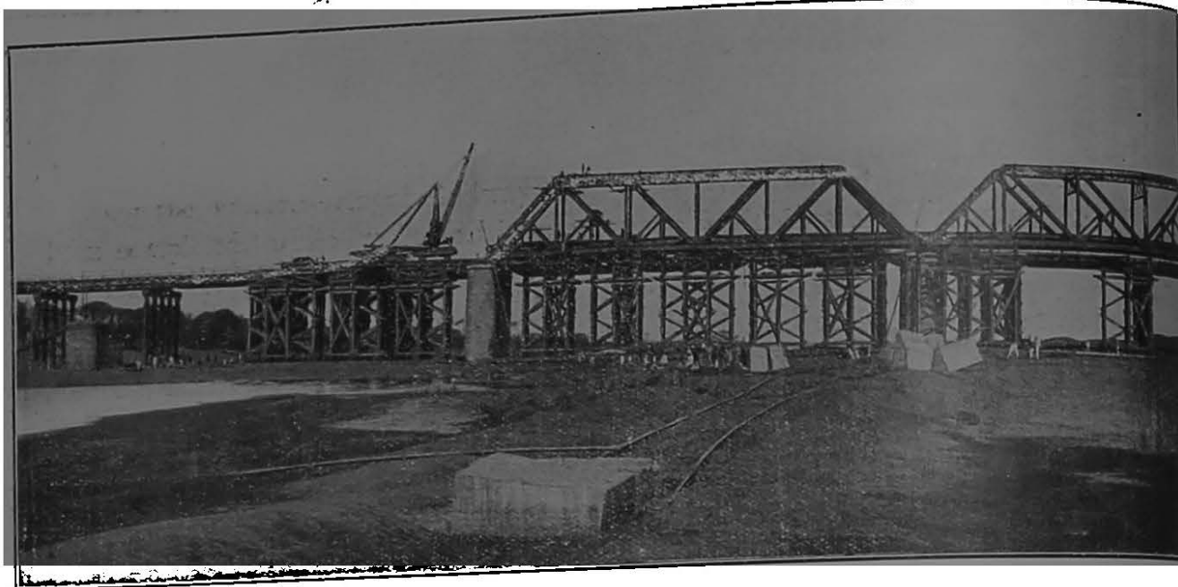
The Rebuilding of the Tapti Bridge—Bombay, Baroda and
