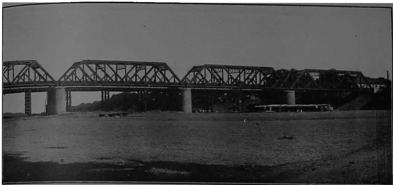
Central India Railway. Ten spans of 187' 6" Double Track.
