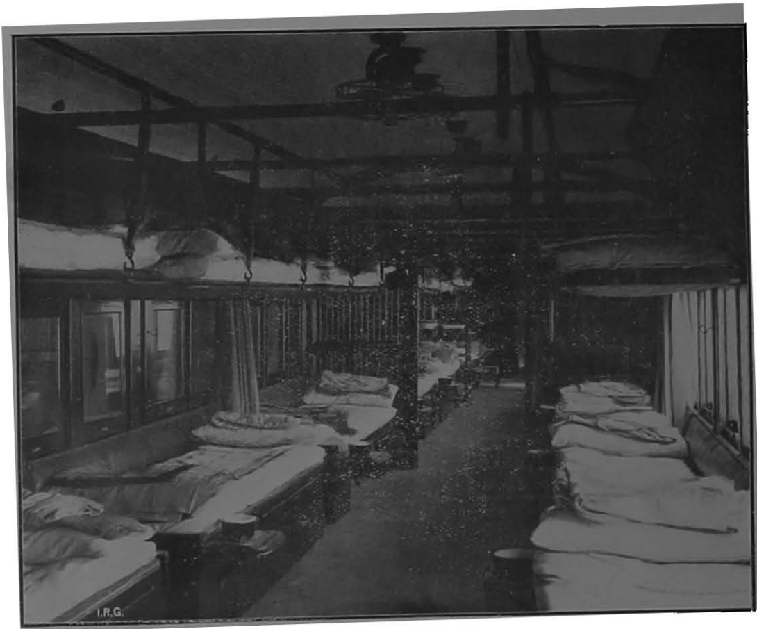
INTERIOR OF AMBULANCE TRAIN.—NORTH WESTERN RAILWAY.
