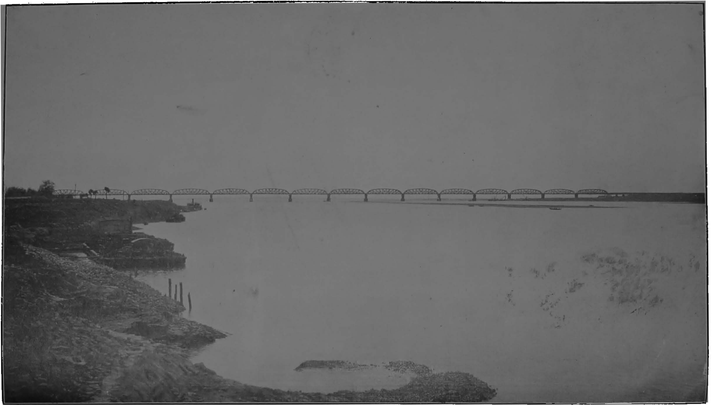
PANORAMIC VIEW OF HARDINGE BRIDGE AS COMPLETED.—UP STREAM OF BRIDGE.
