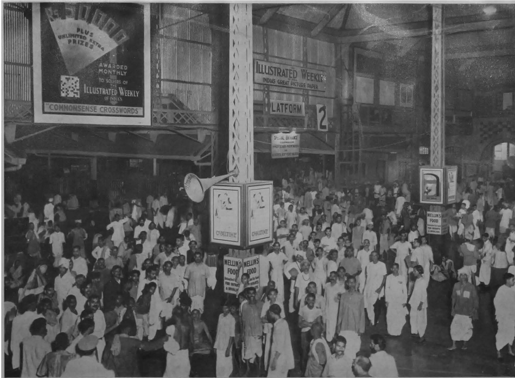
Howrah Station. Main concourse showing loud speakers used for disseminating information to passengers.
