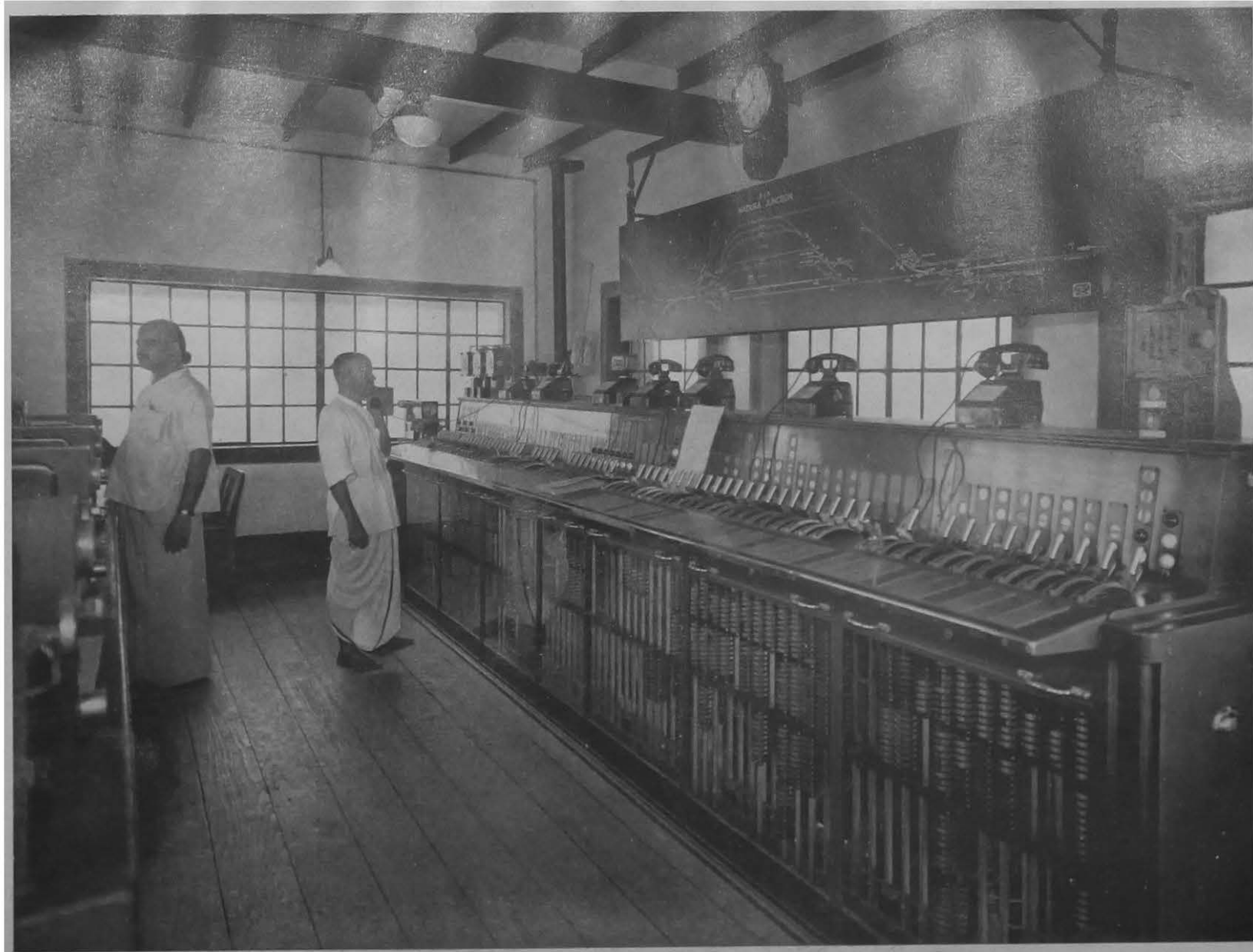
Madura Station. Interior of new power operated signal cabin.
