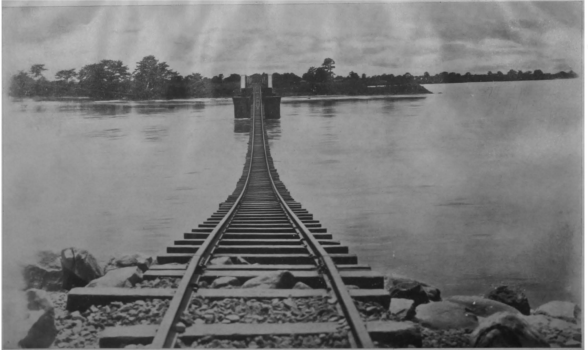
The effect of floods. Breach at Aie Bridge between Bongaigaon and Bijni.
