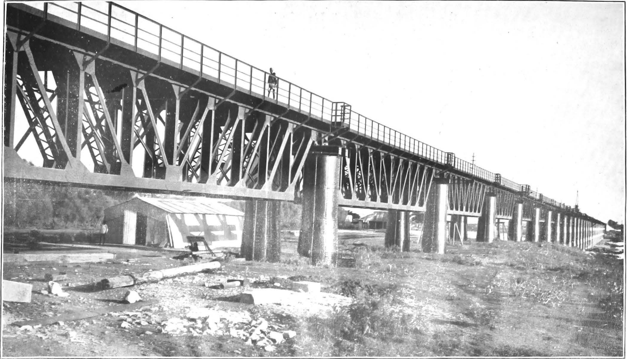
General view of the New Krishna Bridge.
