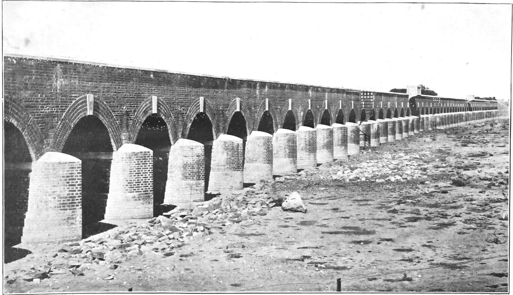
Sone Flood Opening-Bridge (55-12' arches) at mile 357 \frac{1}{2} on the main line.
