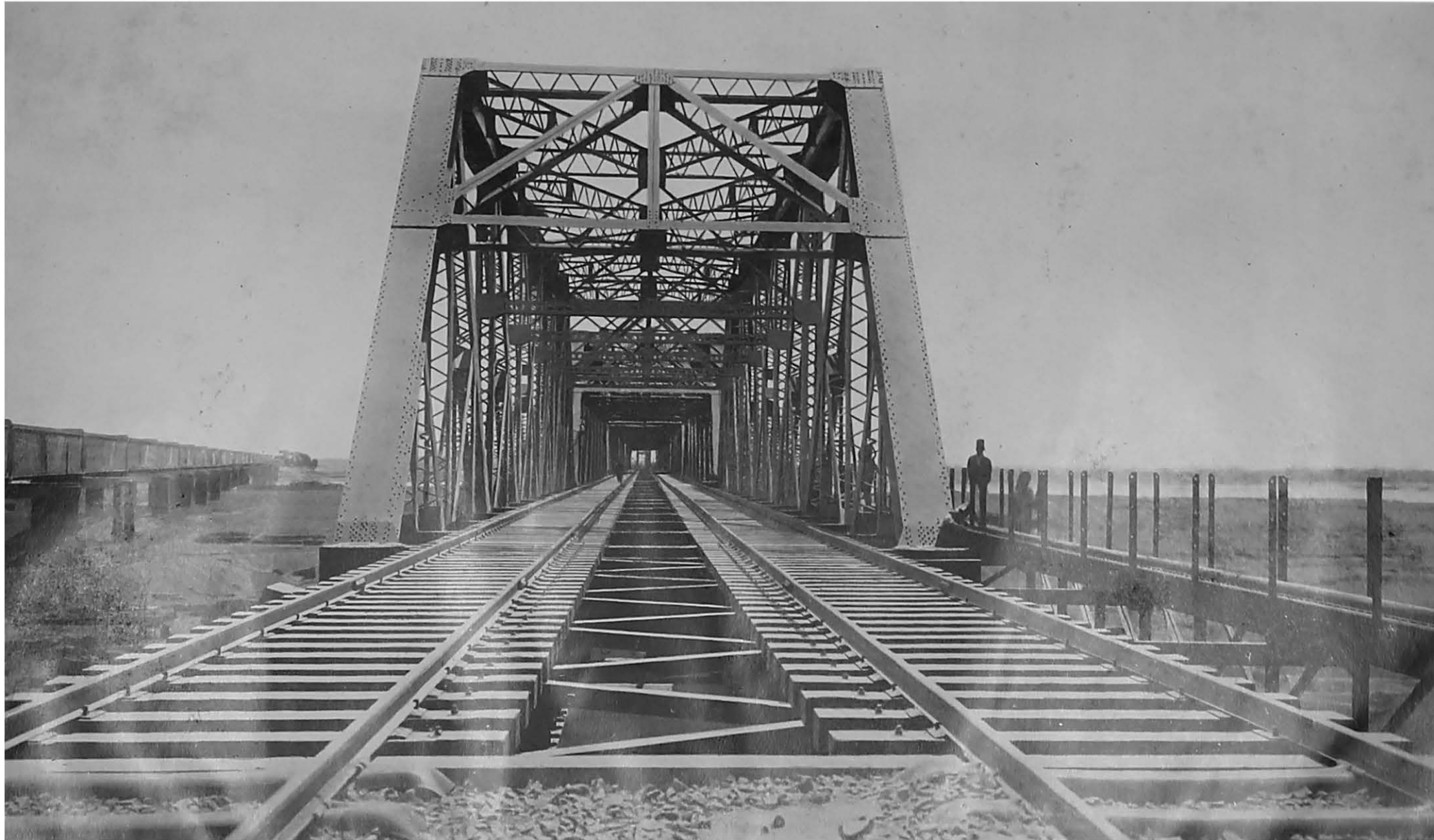
Nerbudda Bridge at Broach. North end-track laid to camber of spans. Existing Bridge on left.
