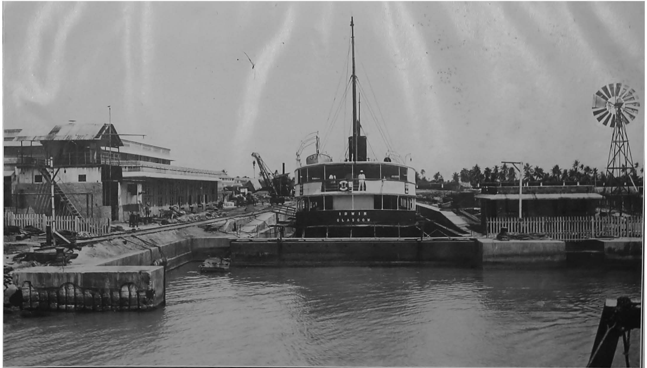
Dry Dock at Mandapam.
