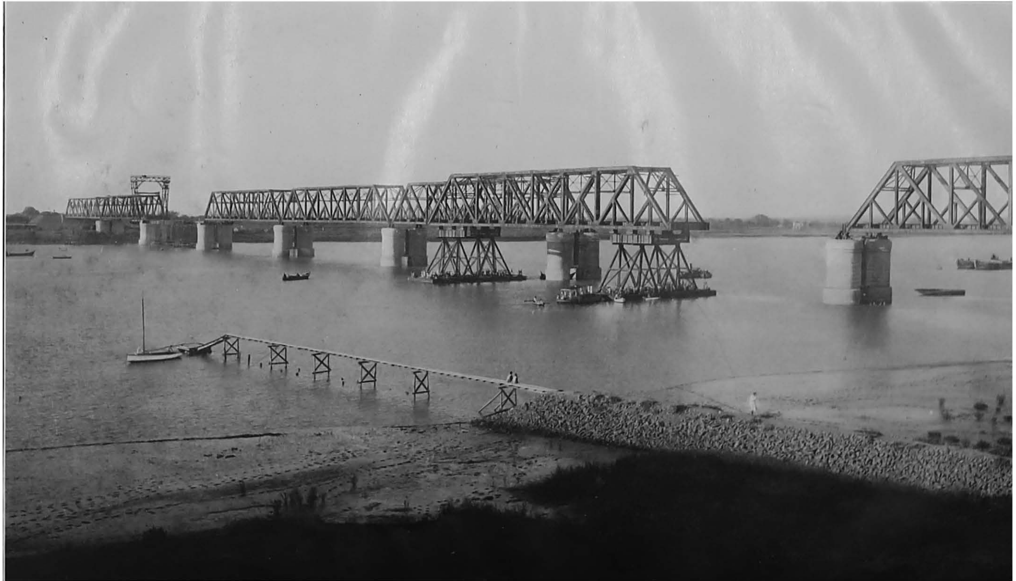
Nerbudda Bridge at Broach. Flotation of Span No. 10.—Fifth and last Flotation.
