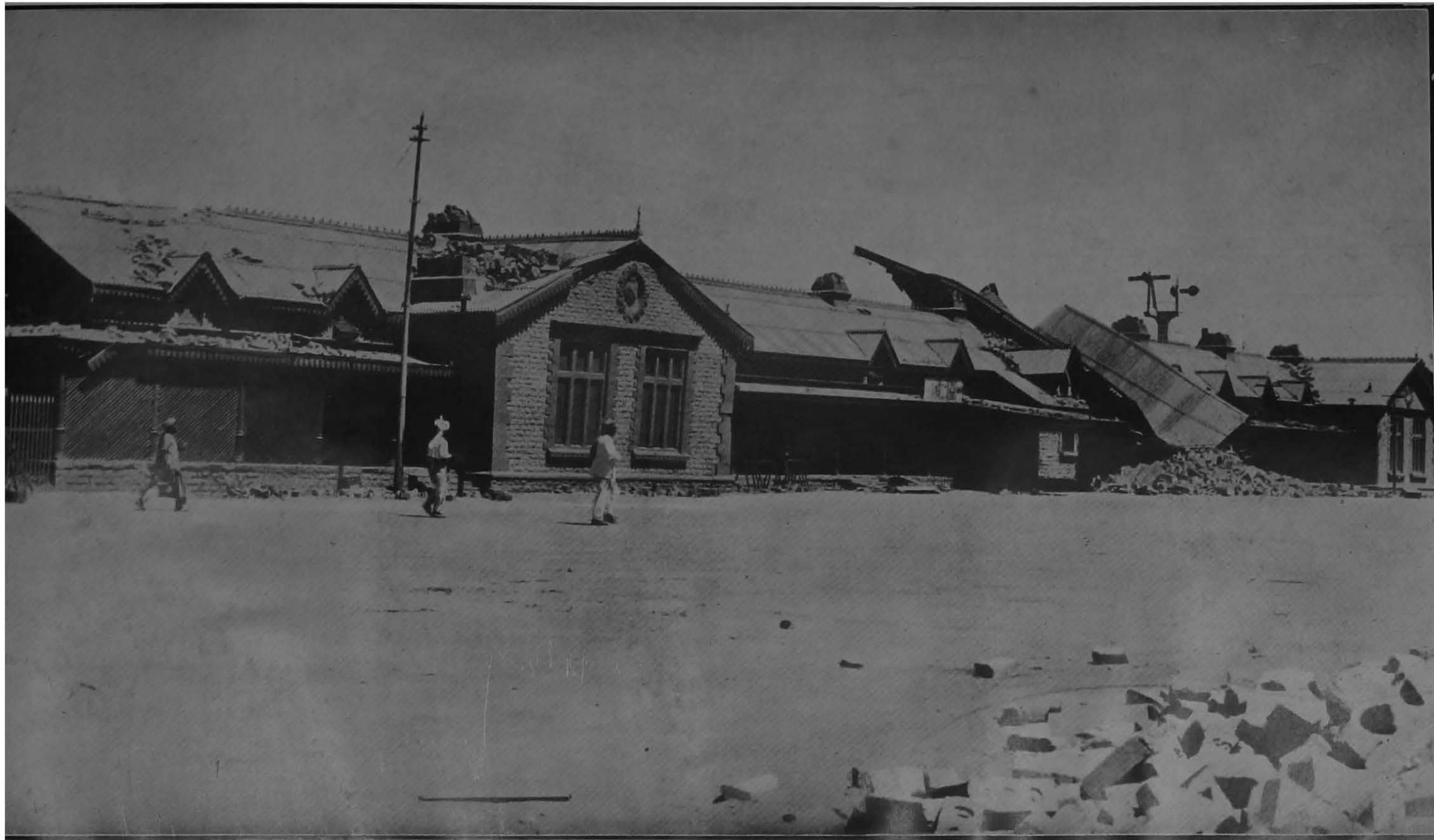
Quetta Railway Station after the earthquake on 31st May 1935.
