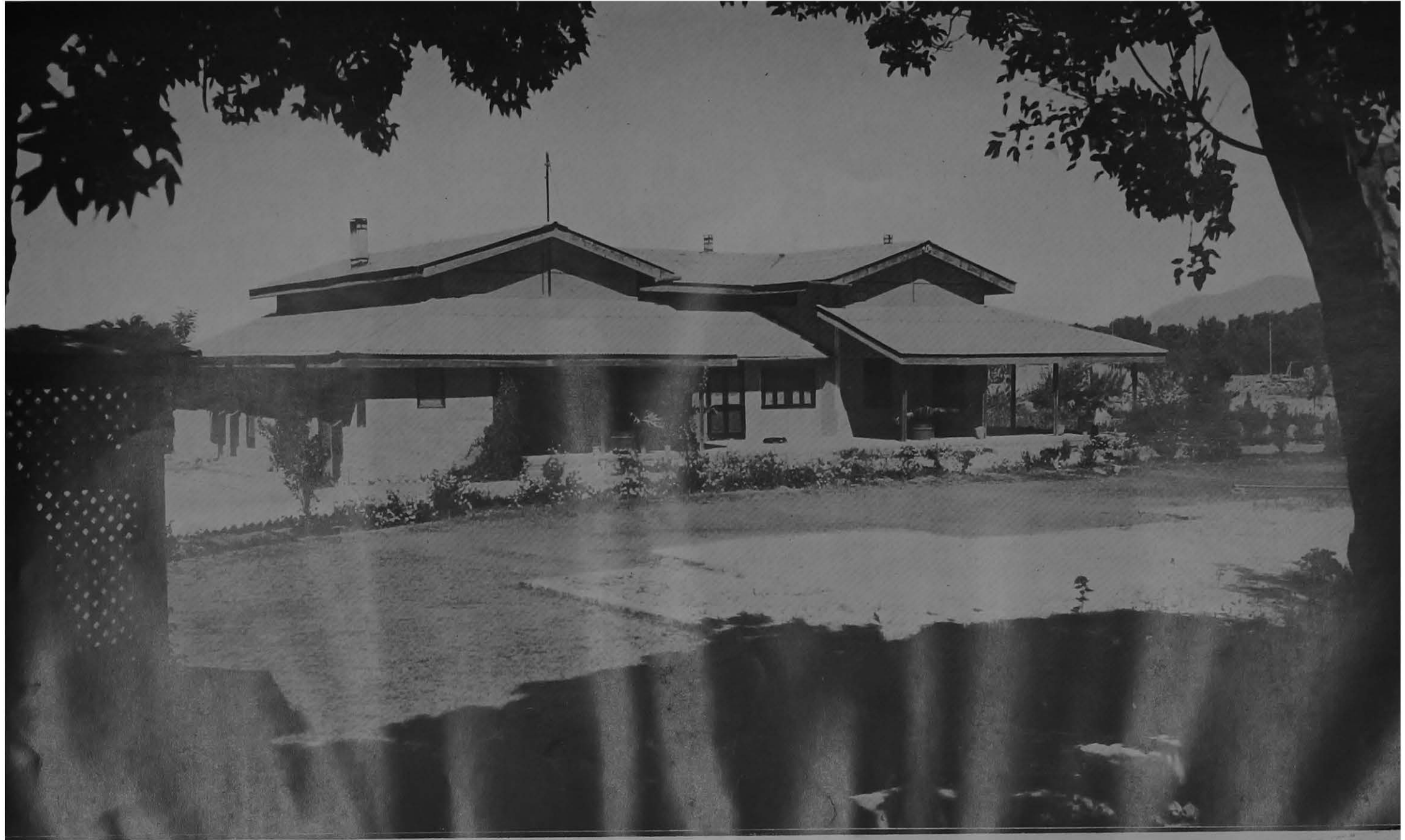
Earthquake-proof Building at Quetta after the earthquake on 31st May 1935.
