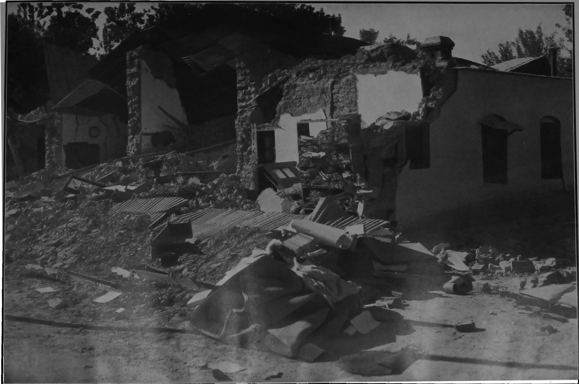
Divisional Superintendent's Office at Quetta after the earthquake on 31st May 1935.
