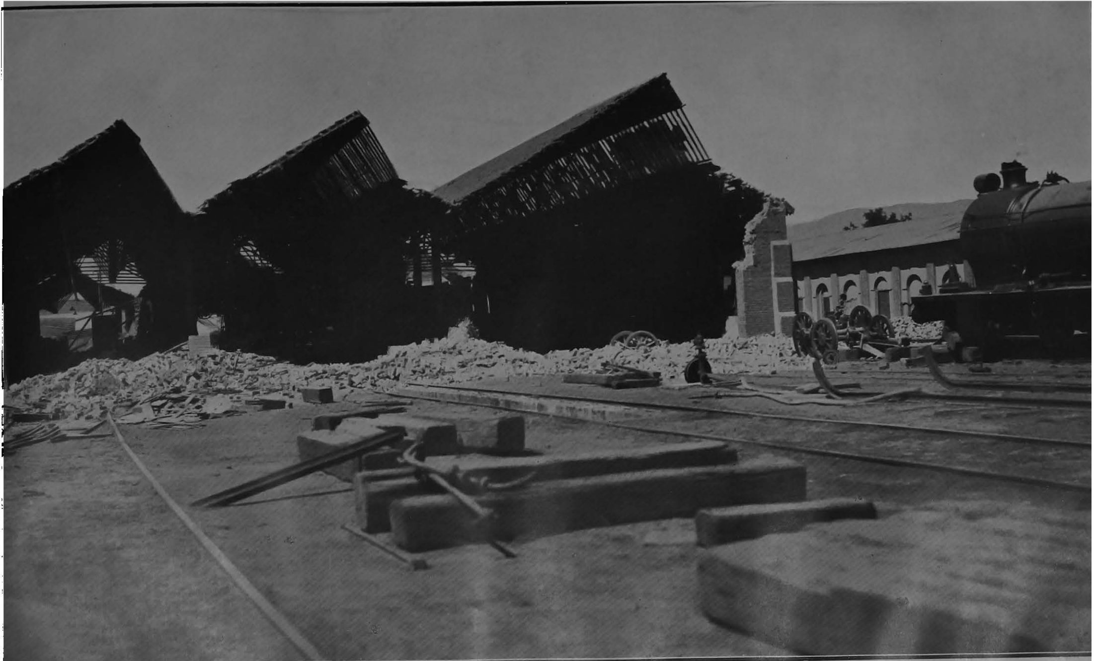
Engine Shed at Quetta after the earthquake on 31st May 1935.
