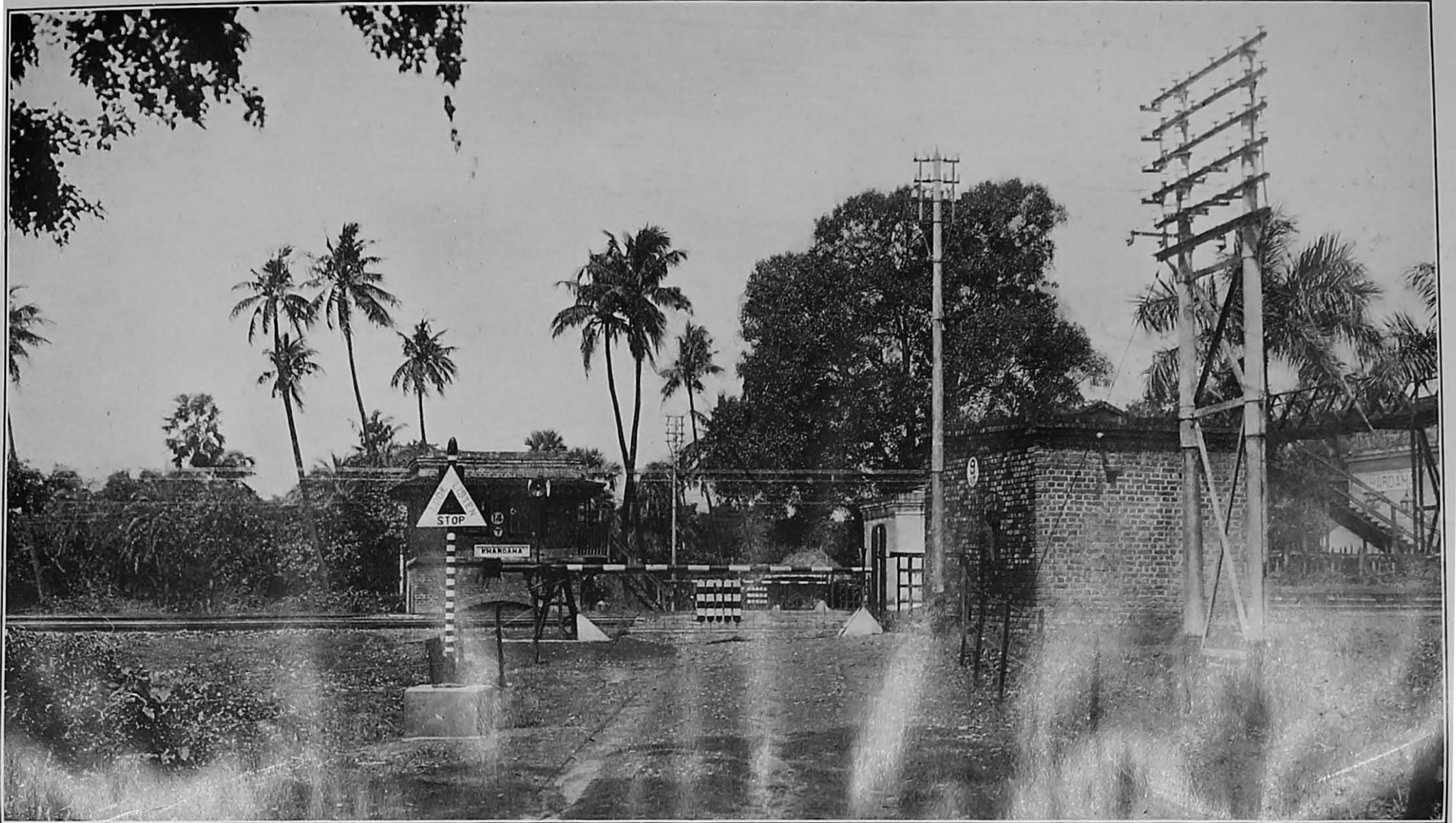
Automatic Level-crossing Barriers at Khardah "Lowered."
