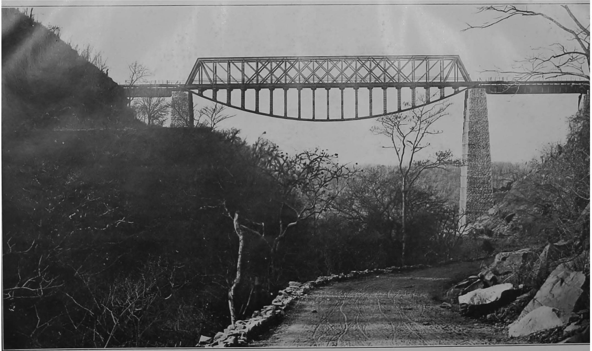
Dhorabhavi Bridge, Guntakal-Bezwada Section—250' span strengthened by underhung bowstring.
