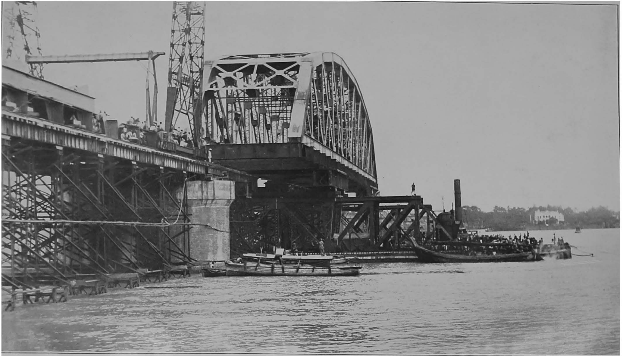
Bally Bridge—350' span being floated from erection bay.
