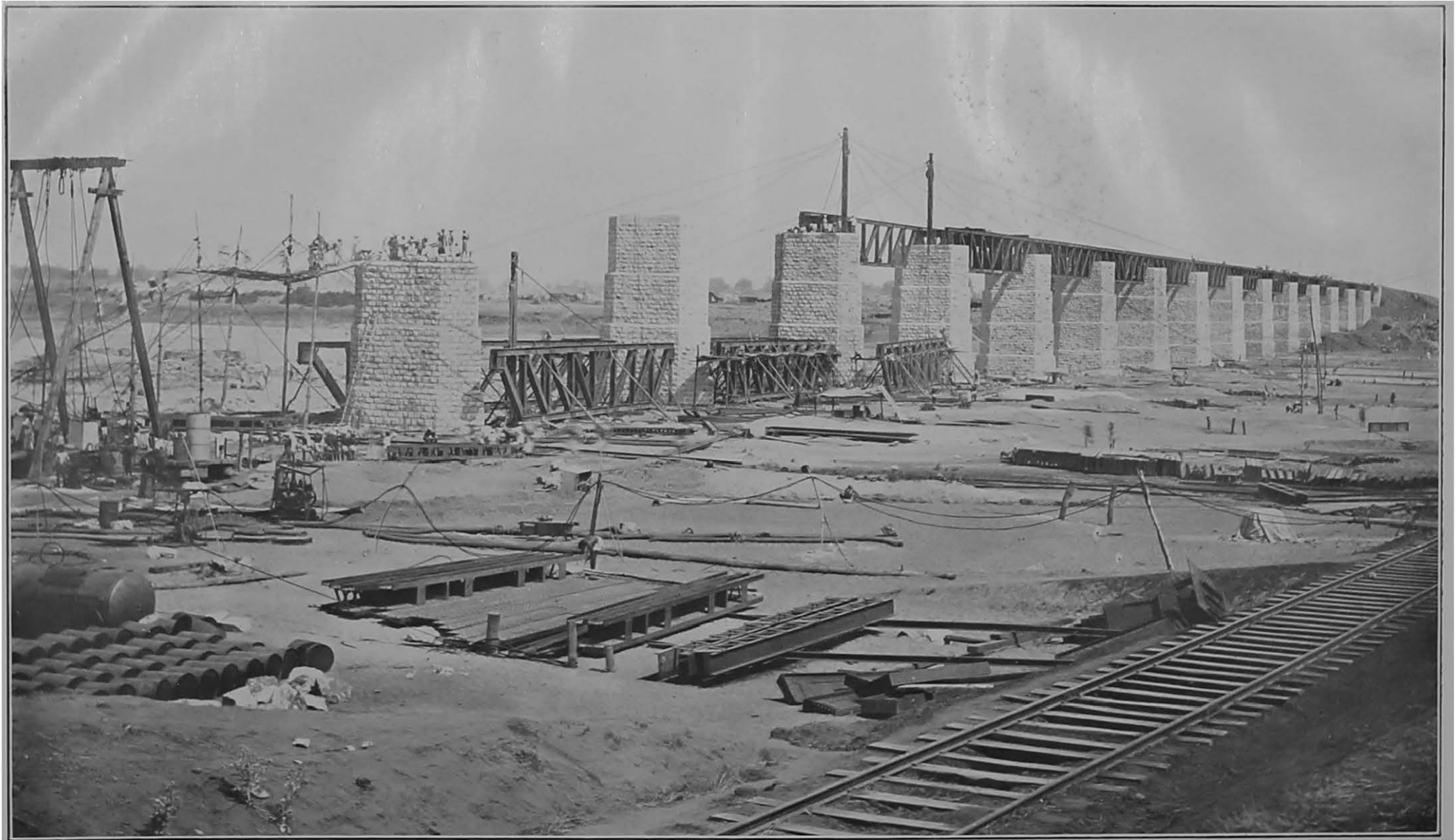
Tel River Bridge in course of construction—Raipur-Vizianagram Section.
