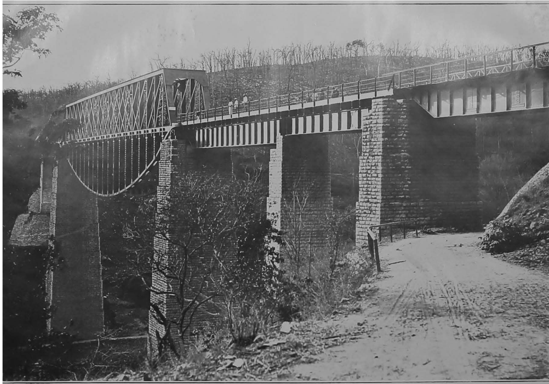
Dhorabhavi Bridge, Guntakal-Bezwada Section—250' span strengthened by underhung bowstring.
